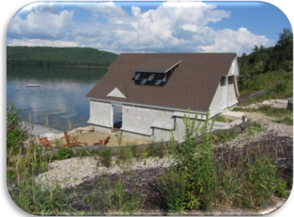
Municipal ordinances are just one tool that can be designed and implemented to protect lake water quality from the effects of watershed development. (Photo: FB Environmental)
