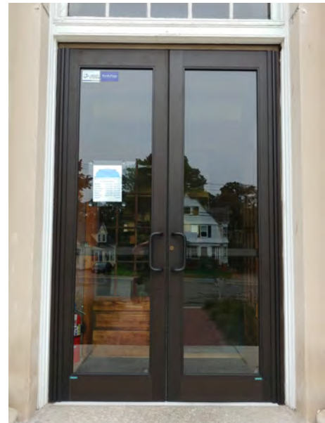
Entry doors at top of south entry stairs.
