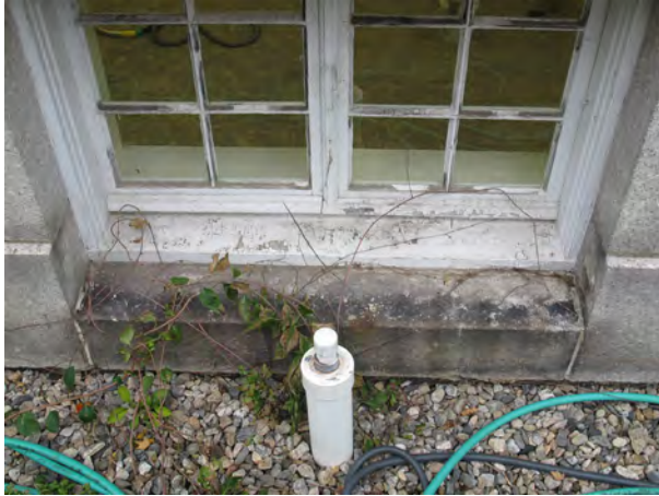
Missing paint on wood elements and glazing.
