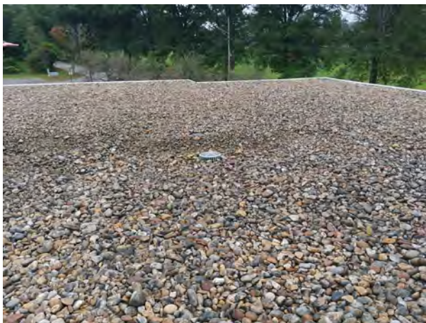
Ballasted roof at 1989 addition.
