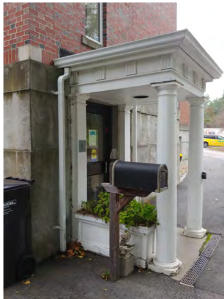
Accessible entry at east elevation, ground level.
