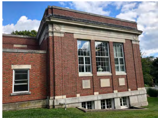
West elevation, south end. Oct. 2018.
