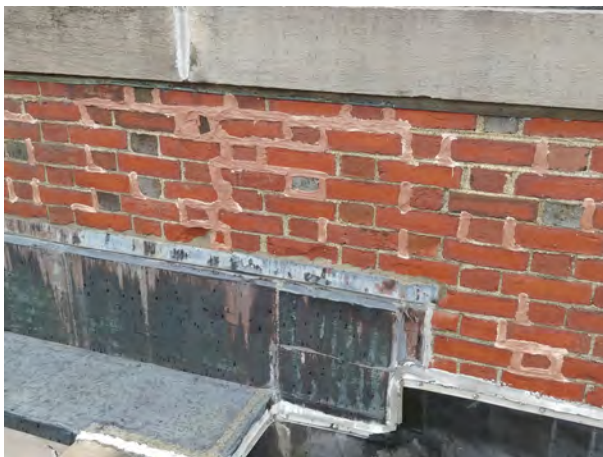
Epoxy compound used for repointing of selected parapet wall areas.
