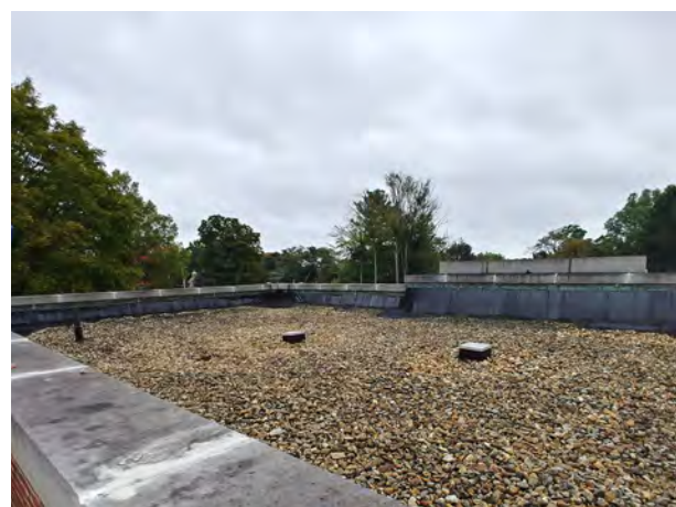
Ballasted roof at 1912 building.
