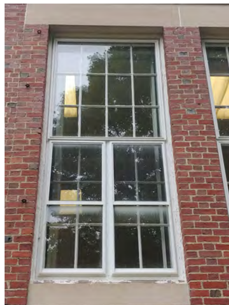
Existing windows at main floor with storm windows.
