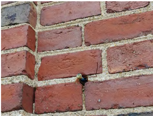
Detail of typical embedded ferrous anchor.
