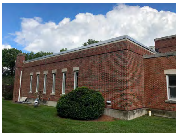
West elevation of 1989 addition. Oct. 2018.
