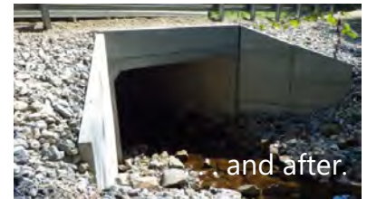
New Hampton Straits Road Culvert
