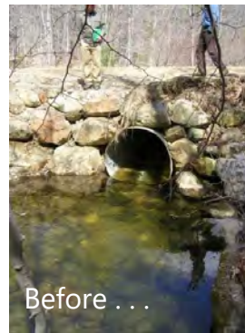
New Hampton Straits Road Culvert
