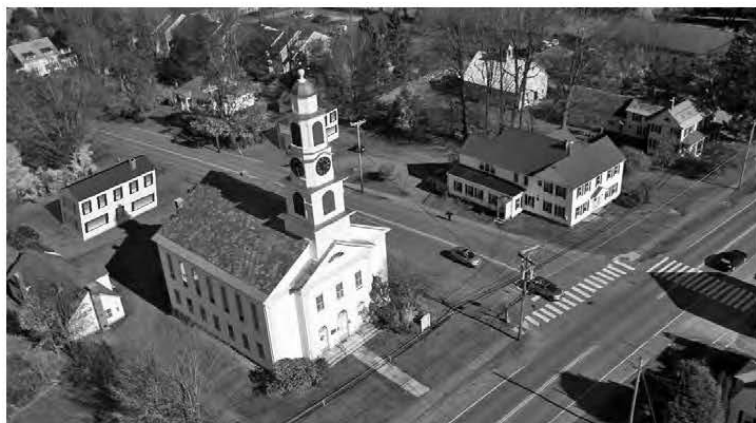
Example of a downtown village where UVLSRPC staff used visuals and local regulations to show what adding housing could look like in this community.
