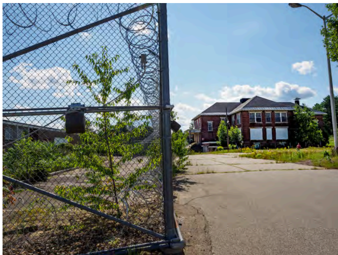
The former Laconia State School property on Aug. 24, 2021. (Alan MacRae | New Hampshire Bulletin)
