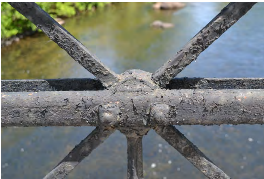
Lattice Corrosion
