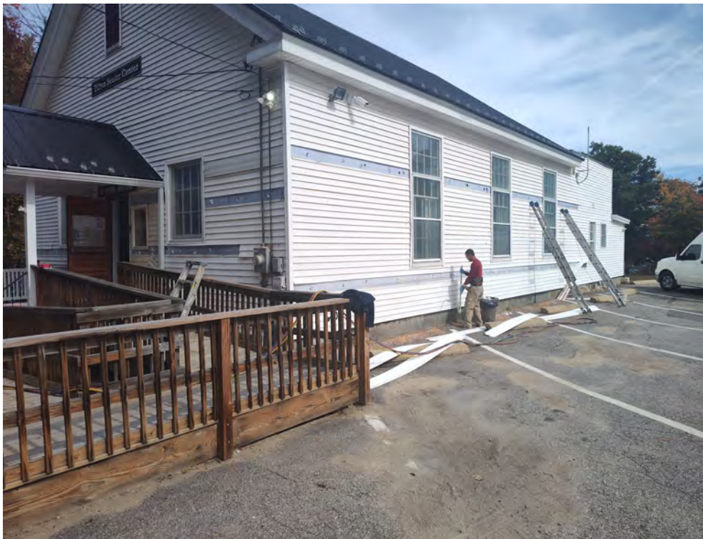
Insulation being installed at the Tilton Senior Center
