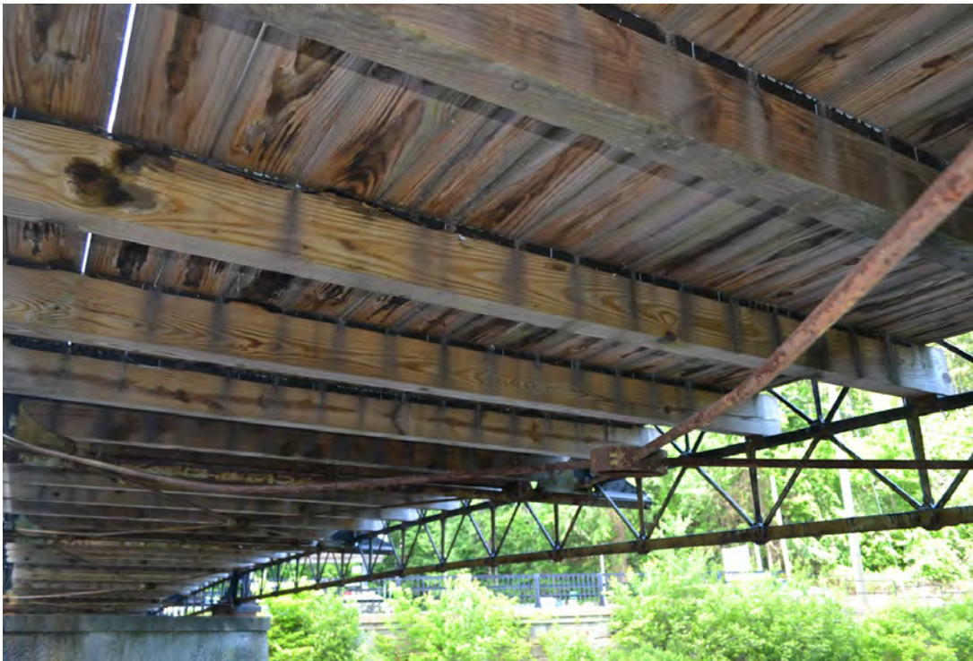
Deck Underside, Diagonal Ties in Compression
