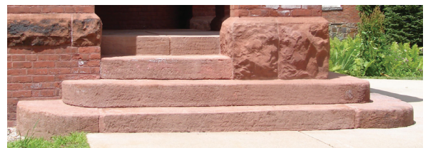
Steps before (TOP) and after repair.
