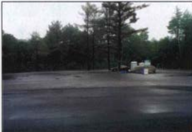
Photo 2: The Site after paving to prevent air infiltration during vacuum extraction. The photo was taken standing where the original house stood and looking north. The pavement was removed and 1,600 poplar trees were planted in this area after the vacuum extraction remedy attained its objectives in 1998.
