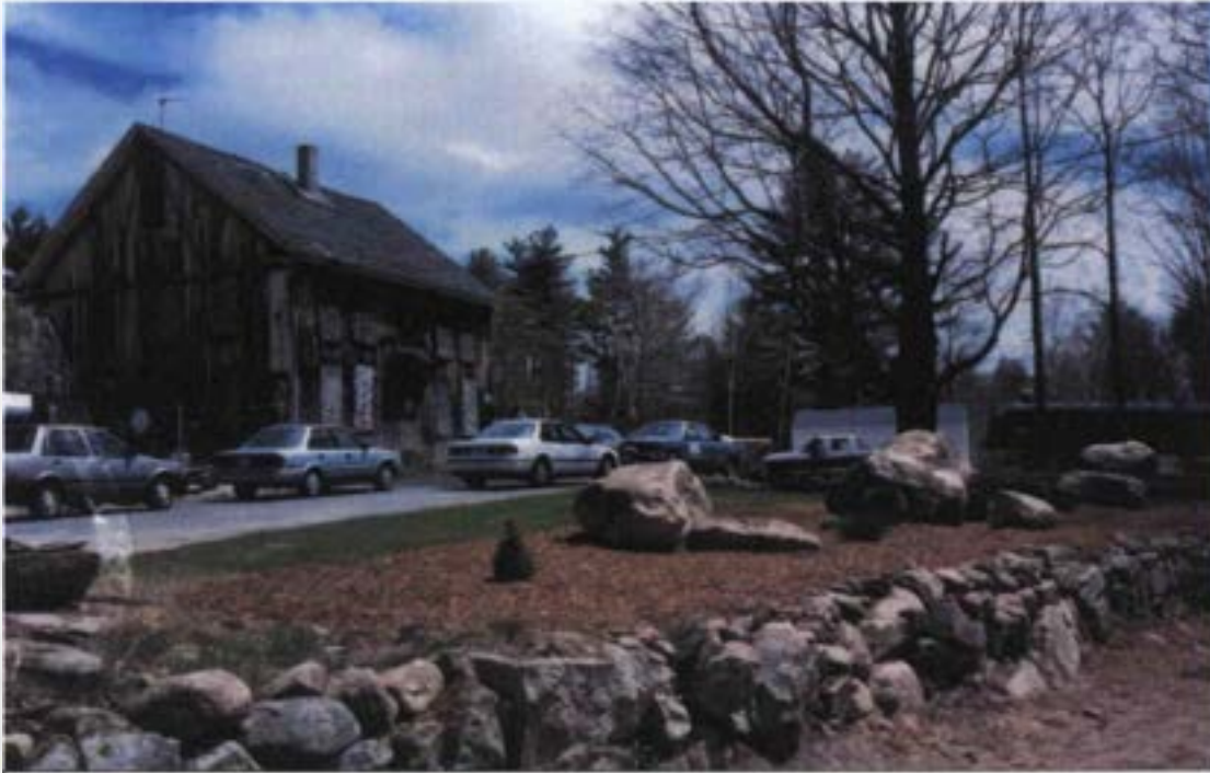
Photo 1: The front of the Site bordering Tibbetts Road and the home, an original post-and-beam, of Alexander Johnson in 1995. The home was demolished as part of the remedy to seal the ground surface for vacuum extraction. The stone wall and large Sugar Maple remain as of 2018.
