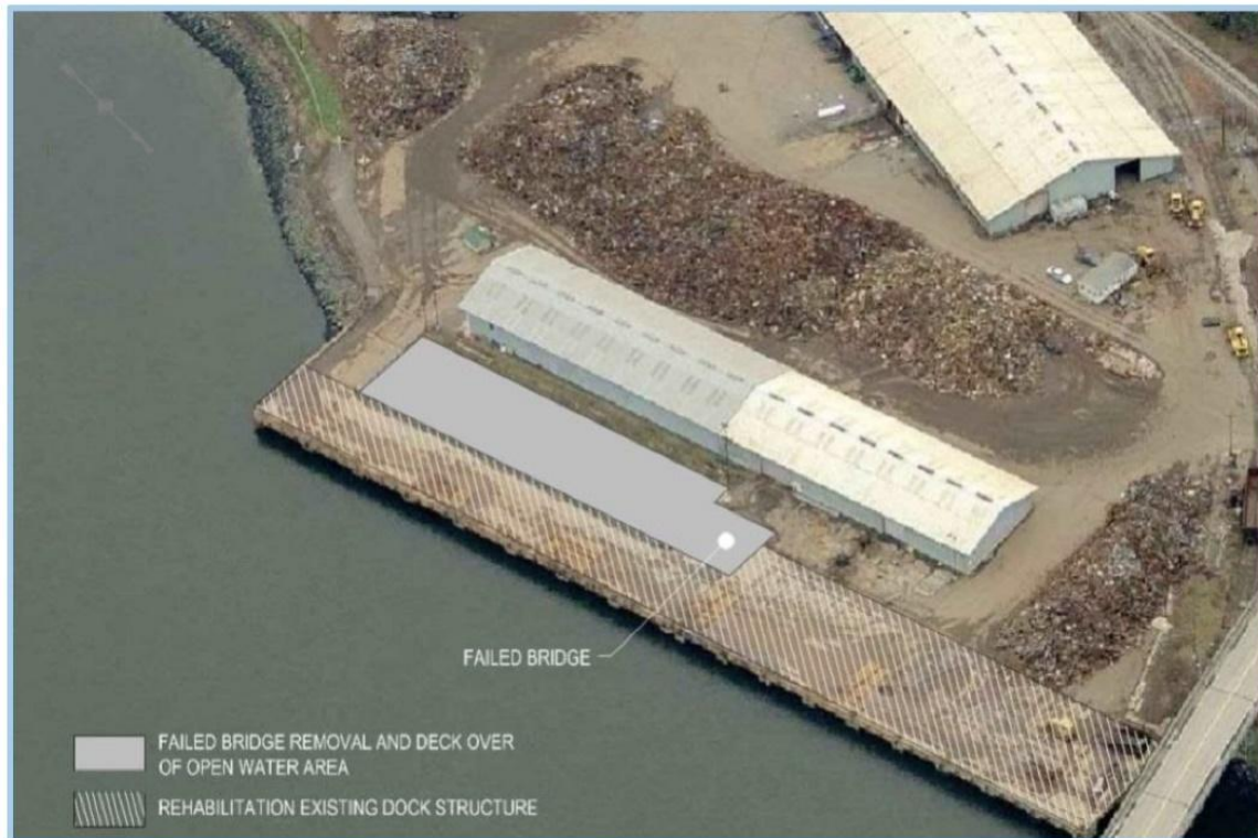
Exhibit 3-5: Port of Portsmouth Main Wharf Rehabilitation Needs 54
