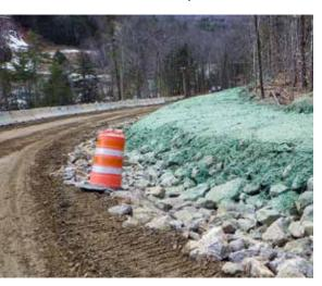
Construction began in December 2017 and will be complete in July 2020. To date the relocation of Houghton Ledge Road is substantially complete with the retaining wall removed and a majority of the steep slope stabilization complete. Drainage replacement and full roadway reconstruction for the 2.1 mile segment will continue through 2018.
