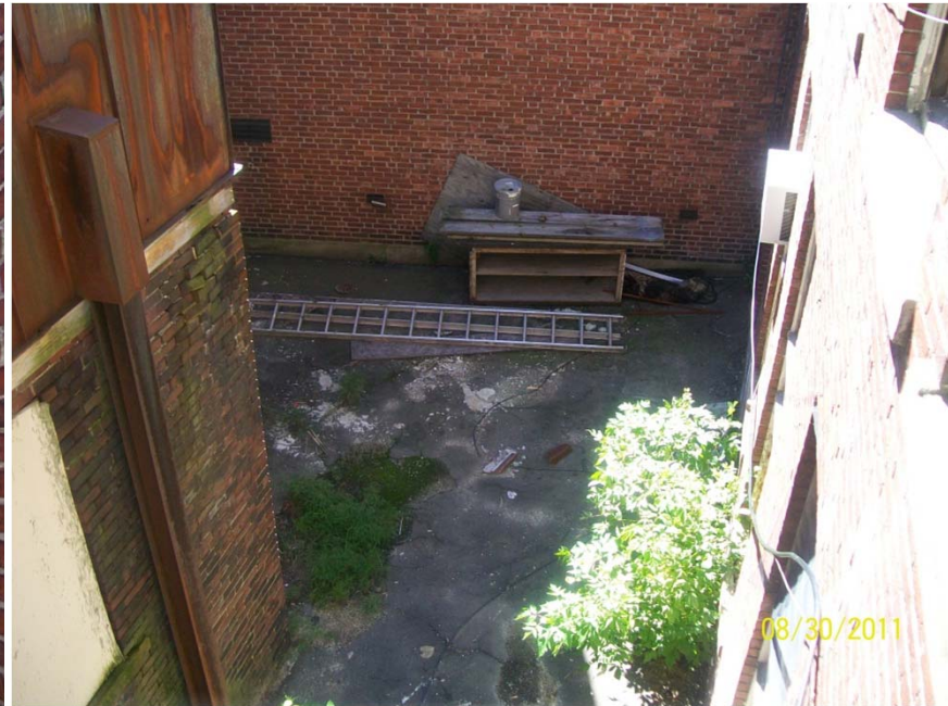
View of the paved courtyard between buildings #1 and #2 (looking east )
