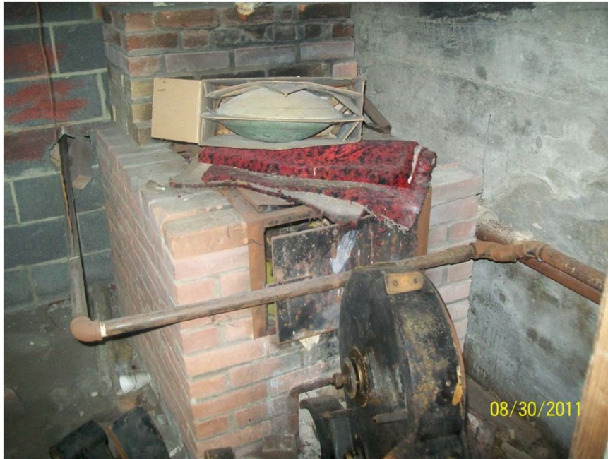
View of former heating system located in basement #3 of building #2
