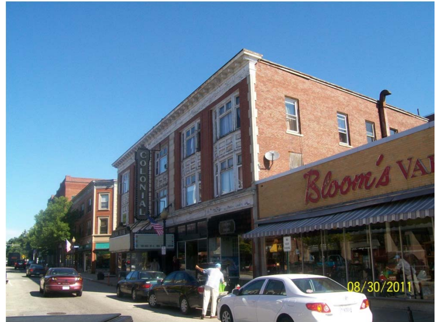
Exterior of subject property building #1 from the corner of Main Street and Hanover Street (looking north)
