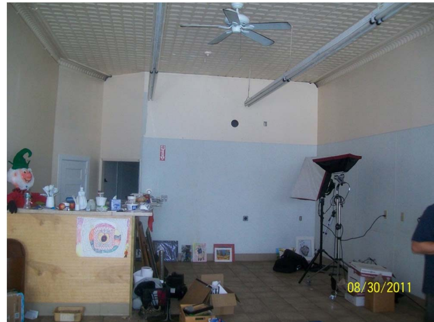
Interior view of representative commercial space in building #2 along Canal Street
