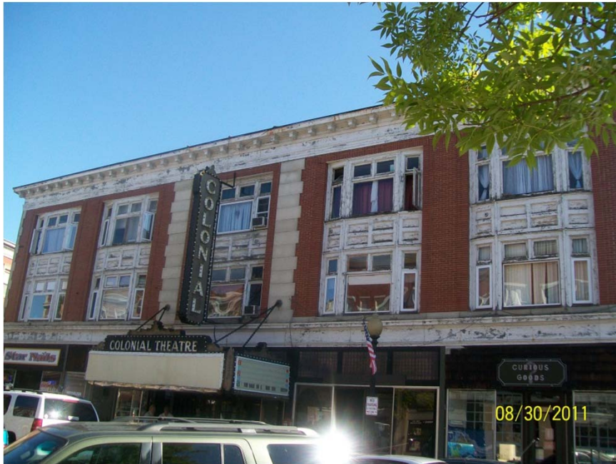
Main Street frontage of subject property building #1 (looking east)
