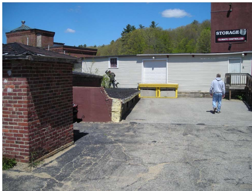
View of west side of the Site parking lot
