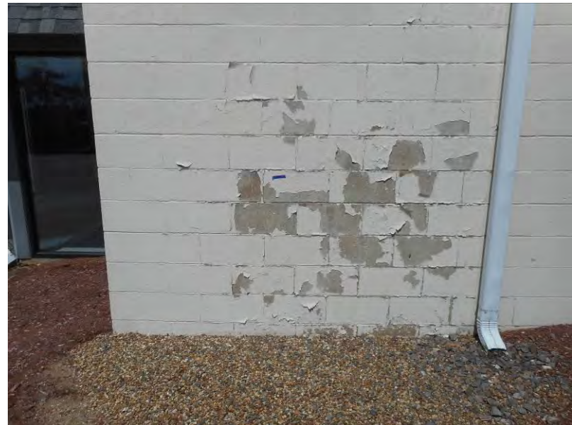
16. Location of CA-PCB-3 collected from white exterior paint on the retail store.
