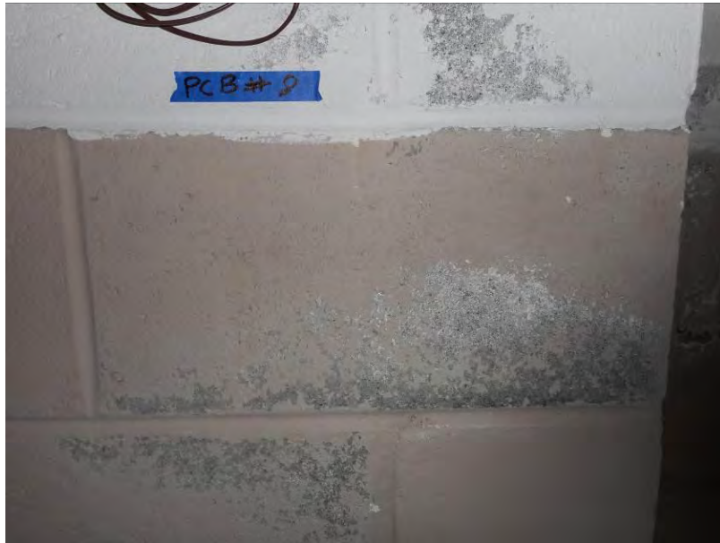
21. Location of CA-PCB-8 collected from beige inter paint of the lower building.
