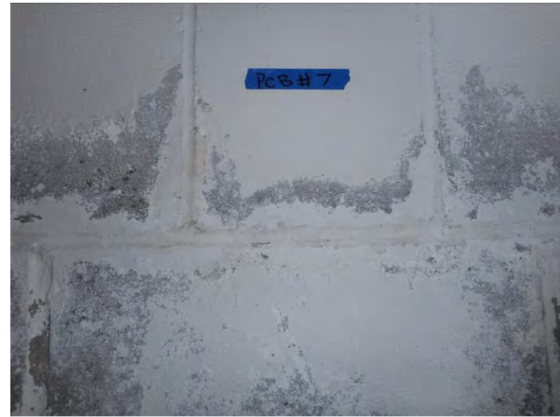
20. Location of CA-PCB-7 collected from white interior paint of the lower building.
