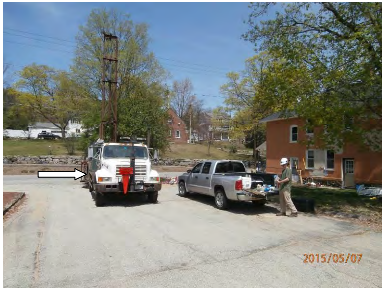
9. Location of CA-SB-9/CA-MW-9 near northeast corner of the retail store.
