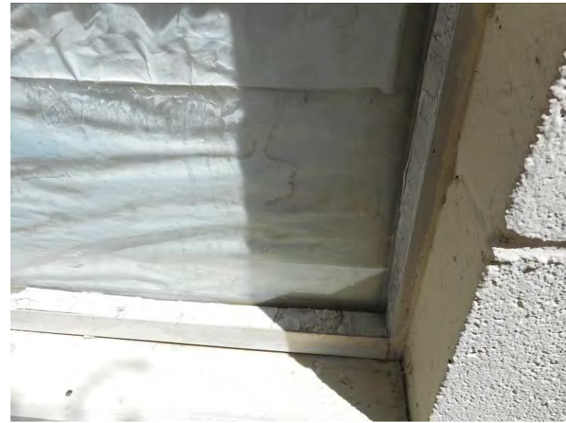
24. Representative photo of ACM window glazing identified at the Site.
