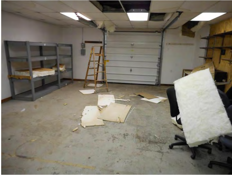
25. Representative photo of ACM ceiling tiles identified at the Site.
