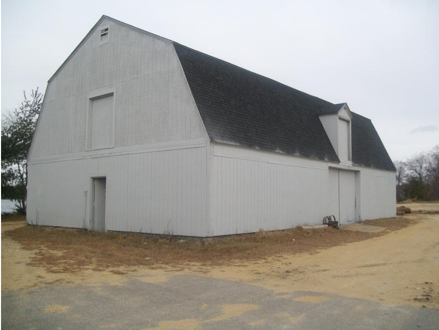
Picture 1 - View of the Horse Barn building looking northwest
