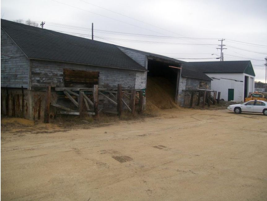
Picture 3 - View of Sand/Salt Shed building looking southeast
