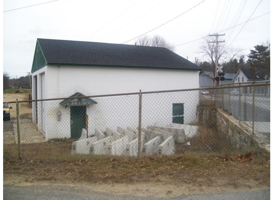
Picture 4 – View of the Vector Shed building looking north
