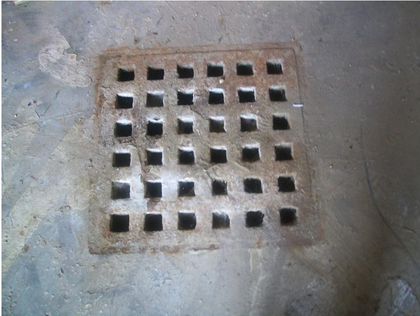
Picture 9 – View of the Vector Shed floor drain structure
