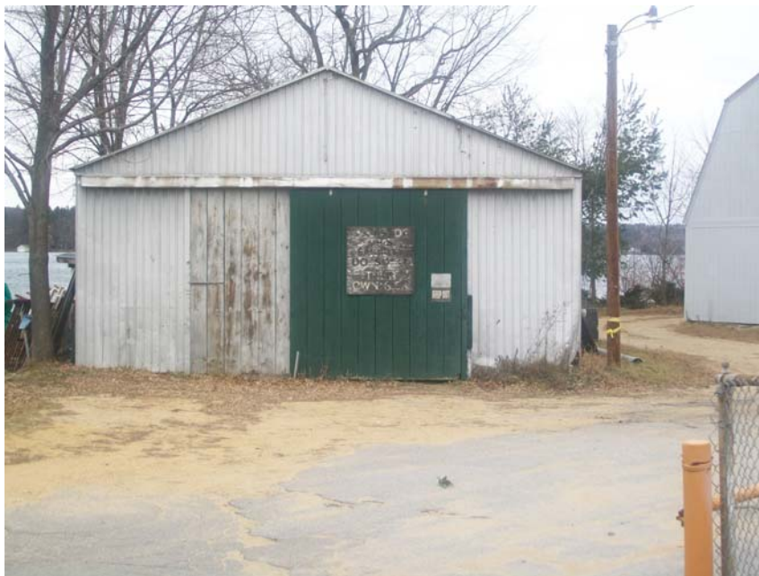
Picture 2 View of the Black- smith Shop build- ing looking west.
