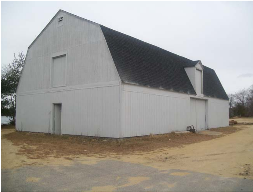
Picture 3 View of the Horse Barn building look- ing northwest.
