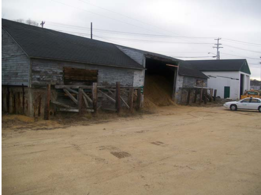
Picture 4 View of the Sand/ Salt Shed building looking southeast.
