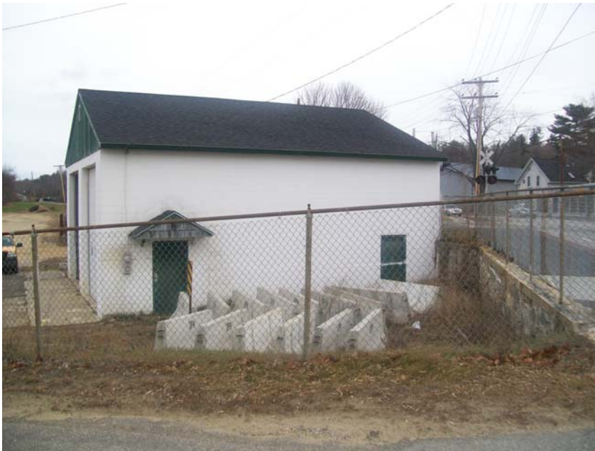
Picture 1 View of the Vector Shed building look- ing north.
