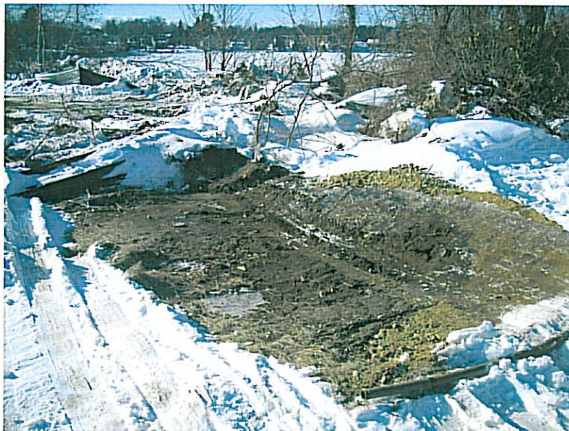
6. View looking to the west of the ground beneath the 9,400-gallon AST following removal on January 12, 2010.
