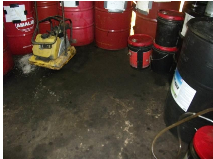
8. Drum storage area within Site building. Note the floor staining.
