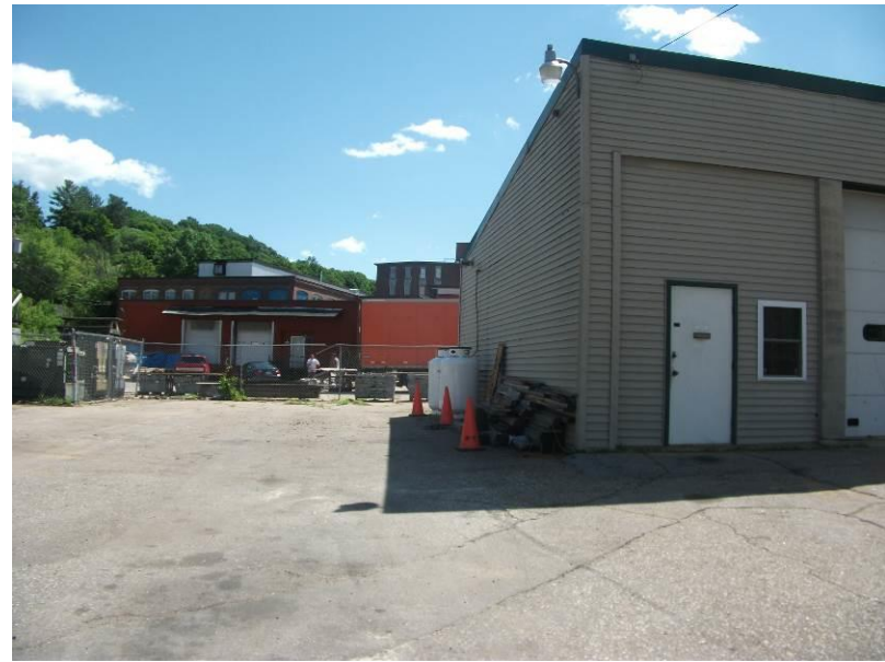
16. Propane tanks outside the northern end of the Site building.
