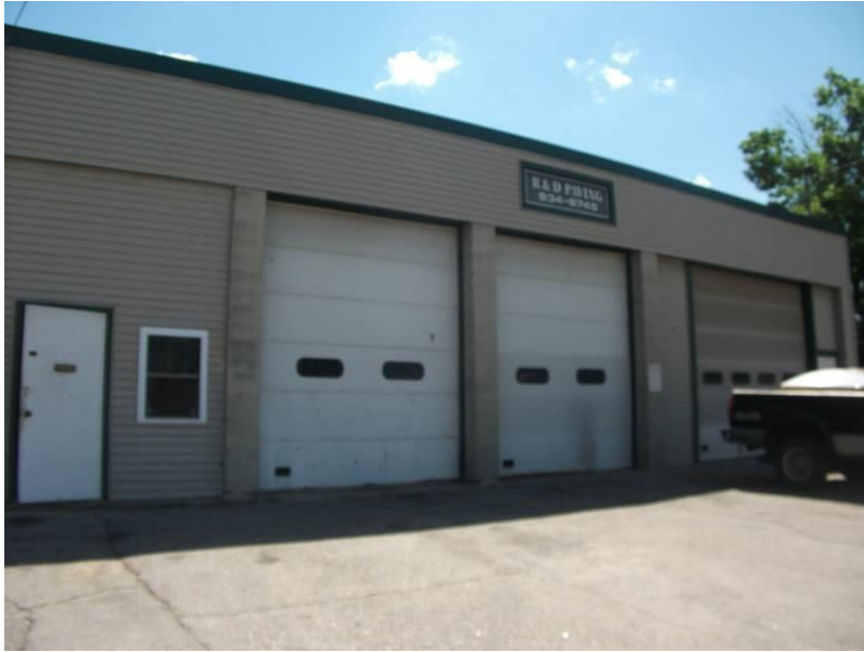
1. View of the Site building looking southeast.
