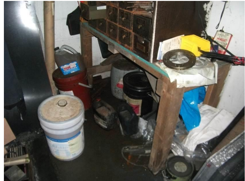
18. View of typical containers within Site building. Note the floor staining.
