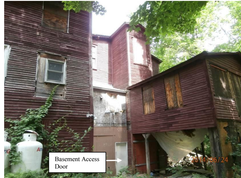
2. Image showing the Site building and basement access door looking north.
