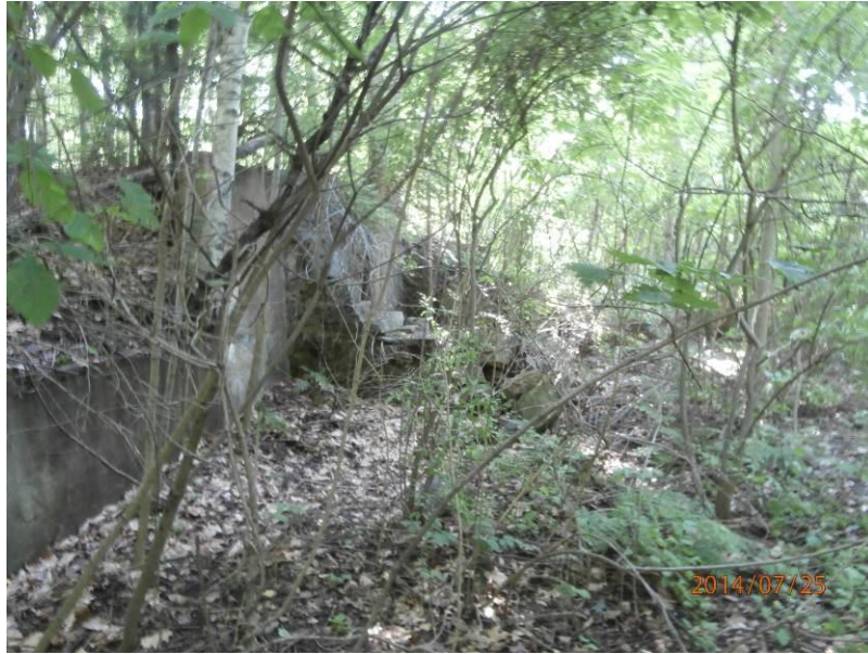
29. Remnants of stone and concrete foundation of historical foundry looking east.
