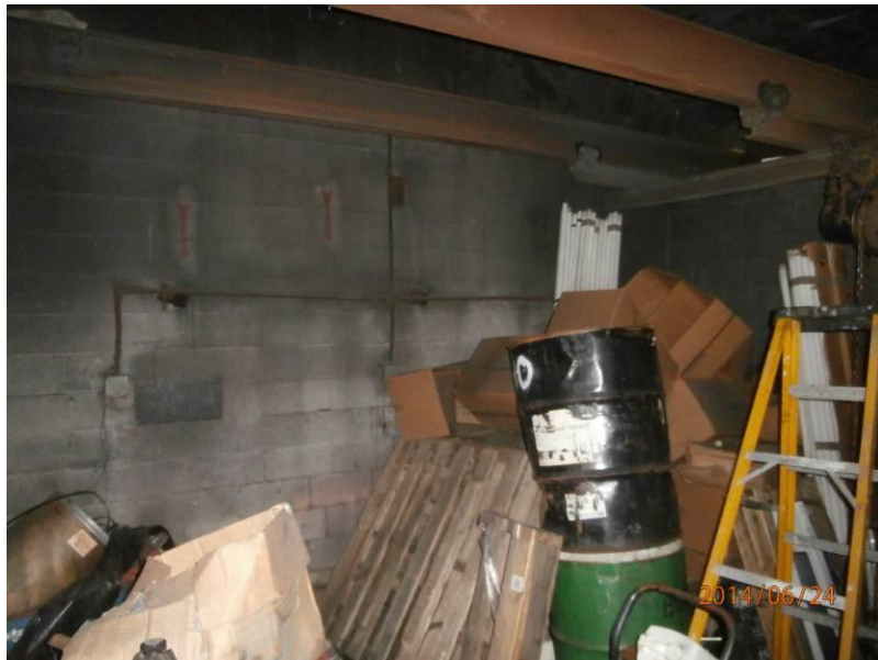
11. Image showing miscellaneous debris, including waste fluorescent bulbs typical of the Site building interior.
