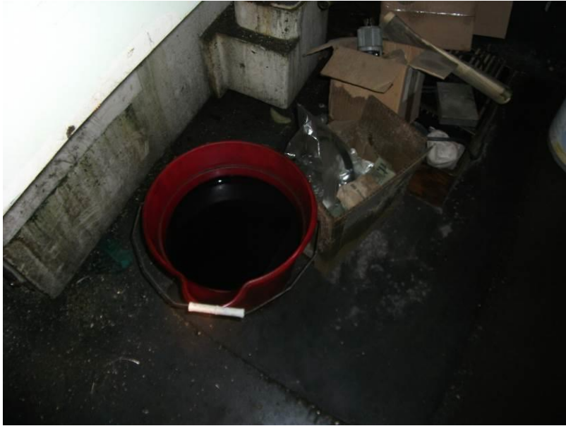
13. View of typical containers within Site building. Note the floor staining.
