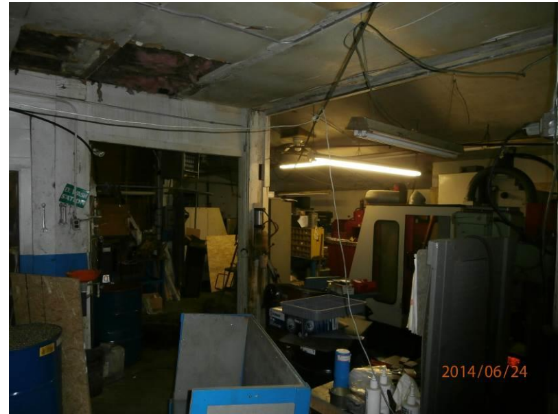
6. Image showing typical remnant equipment within the building.
