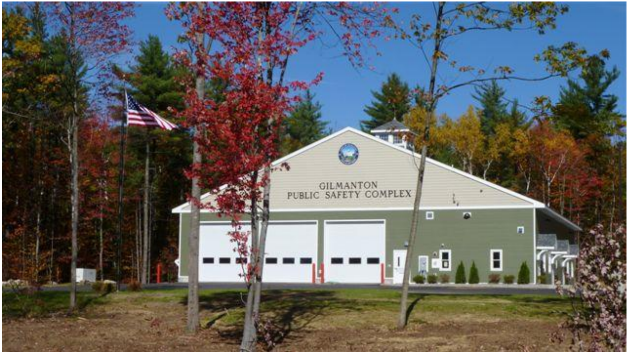
Gilmanton Public Safety Complex
