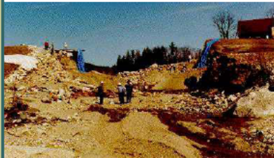
Alton dam breach, 1996
