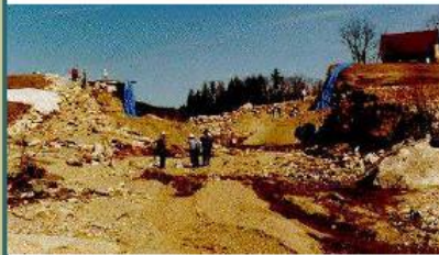
Alton dam breach, 1996
