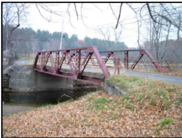
Braley Road Bridge built c1927
