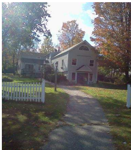
Locust Cottage – rear addition
