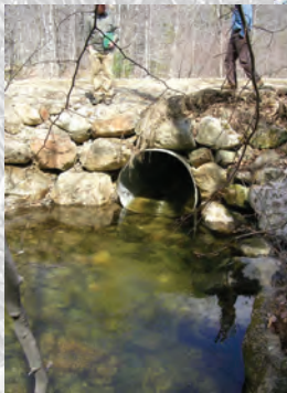
Culverts, Straits Road, New Hampton old and new
