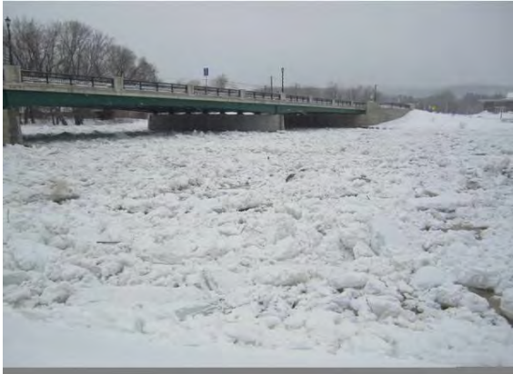
March 2011 Ice Jam at NH Route 175A bridge across the Pemigewasset River
