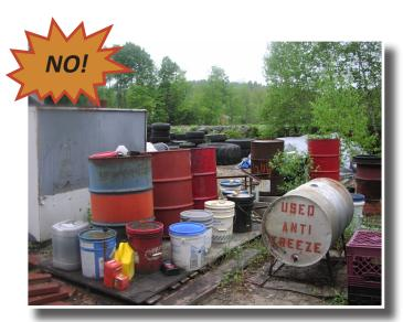
Antifreeze containers are in poor condition and some are open. There is no secondary containment to catch spills and leaks. These containers are not stored on concrete or other impervious surfaces to prevent leaks into the environment. They are exposed to the weather and should be under a roof.
