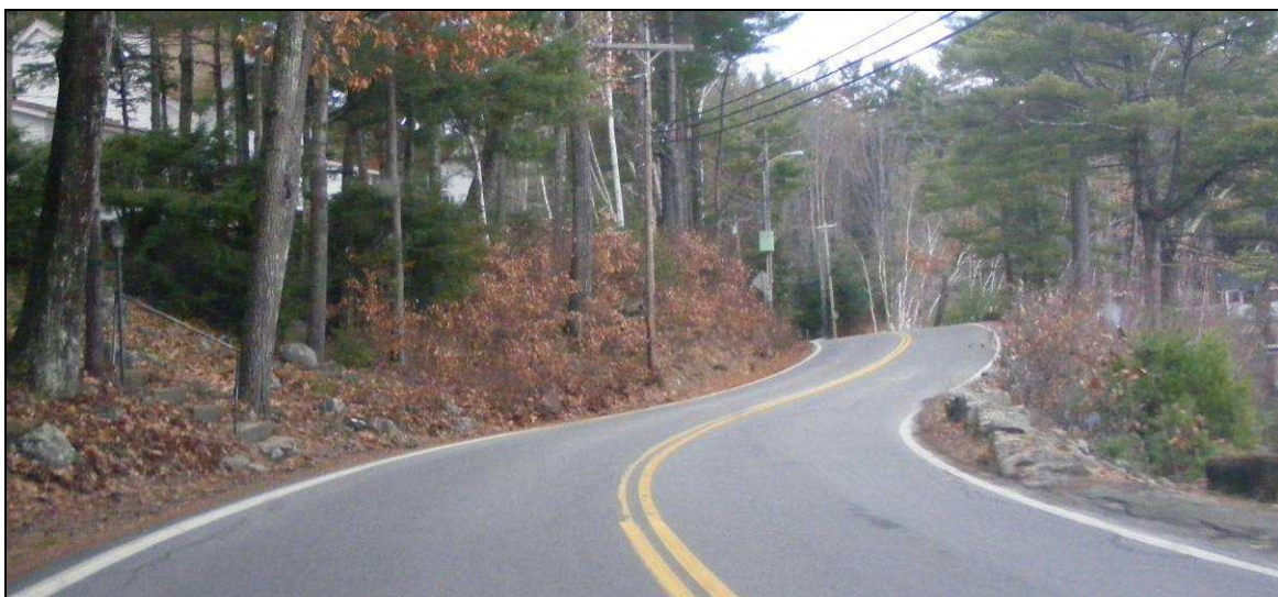
NH Route 113 Priority Area – Narrow Shoulders, Horizontal Curves, Limited Sight Distance
