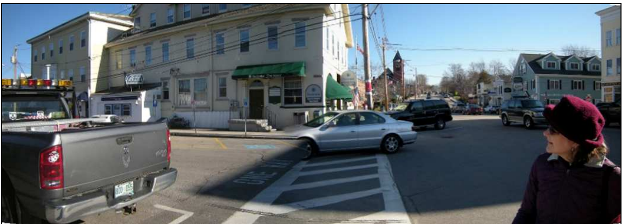
Main Street / Depot Street Intersection – note dangerous parking configuration
