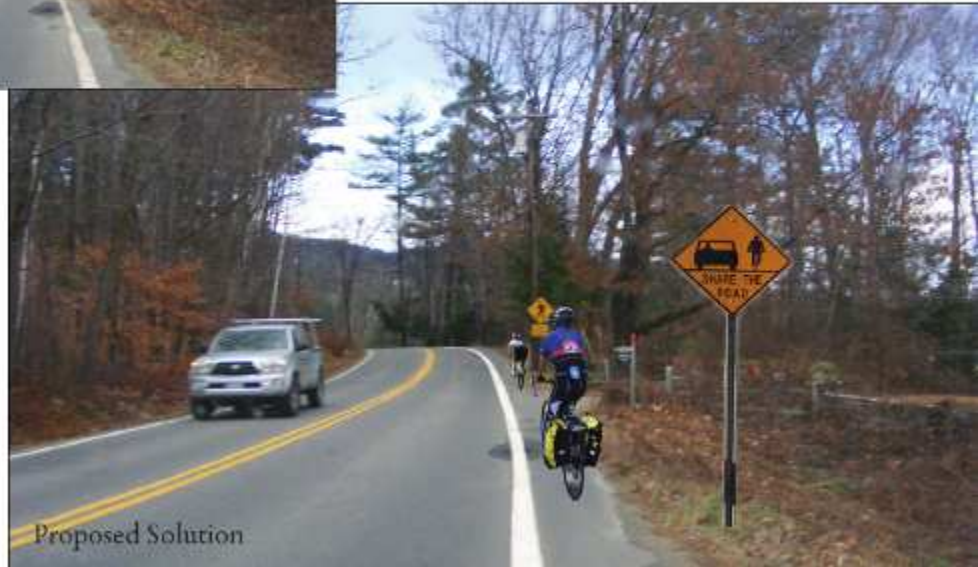
Conceptual rendering of a lane width modification along NH Route 113 in Holderness. Existing 11½ - 12 foot lane is shown above. Proposed improvement with 10½ - 11 foot lanes using existing pavement is shown below, with added ‘Share the Road’ signage.
