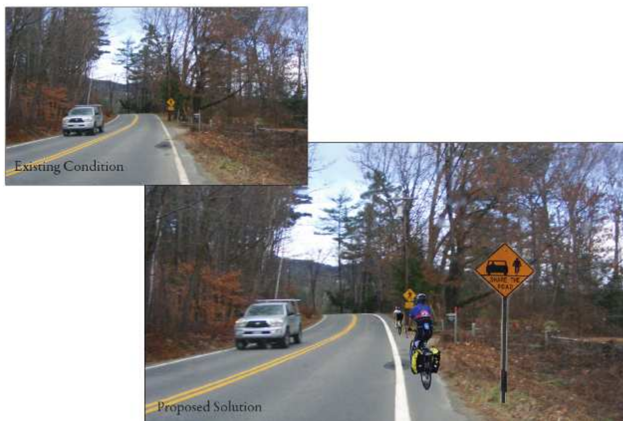
Fig. 21 - Conceptual rendering of a lane width modification along NH Route 113 in Holderness. Existing 11½ - 12 foot lane is shown above. Proposed solution with 10½ - 11 foot lane using existing pavement is shown below, with added Share the Road signage.
