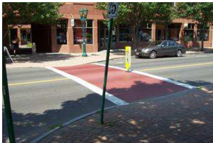
Fig. 26 – Mid-block crossing with bump-outs and a high visibility bollard
