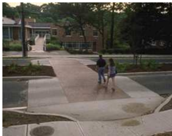
Fig. 25 – Mid-block speed tables can be a good solution for high volume boulevards with high pedestrian volumes, like US Route 3 in Meredith
