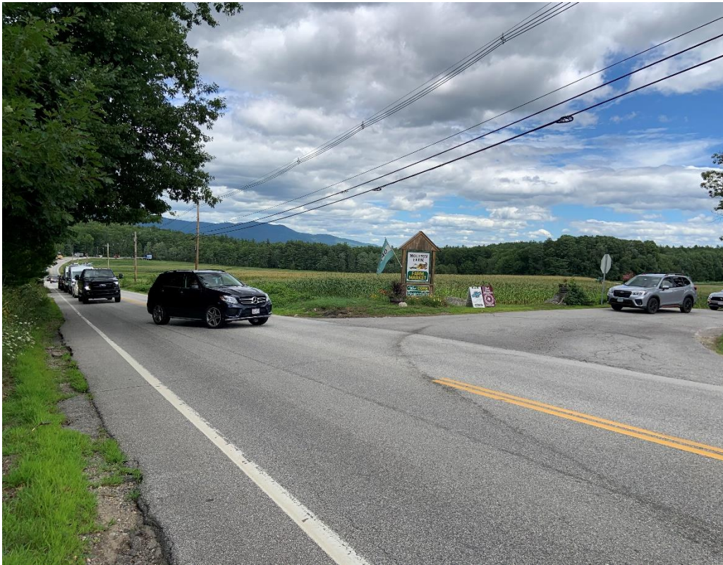
3-A NH Route 25 at Quarry Road facing east. Note inadequate shoulder.
