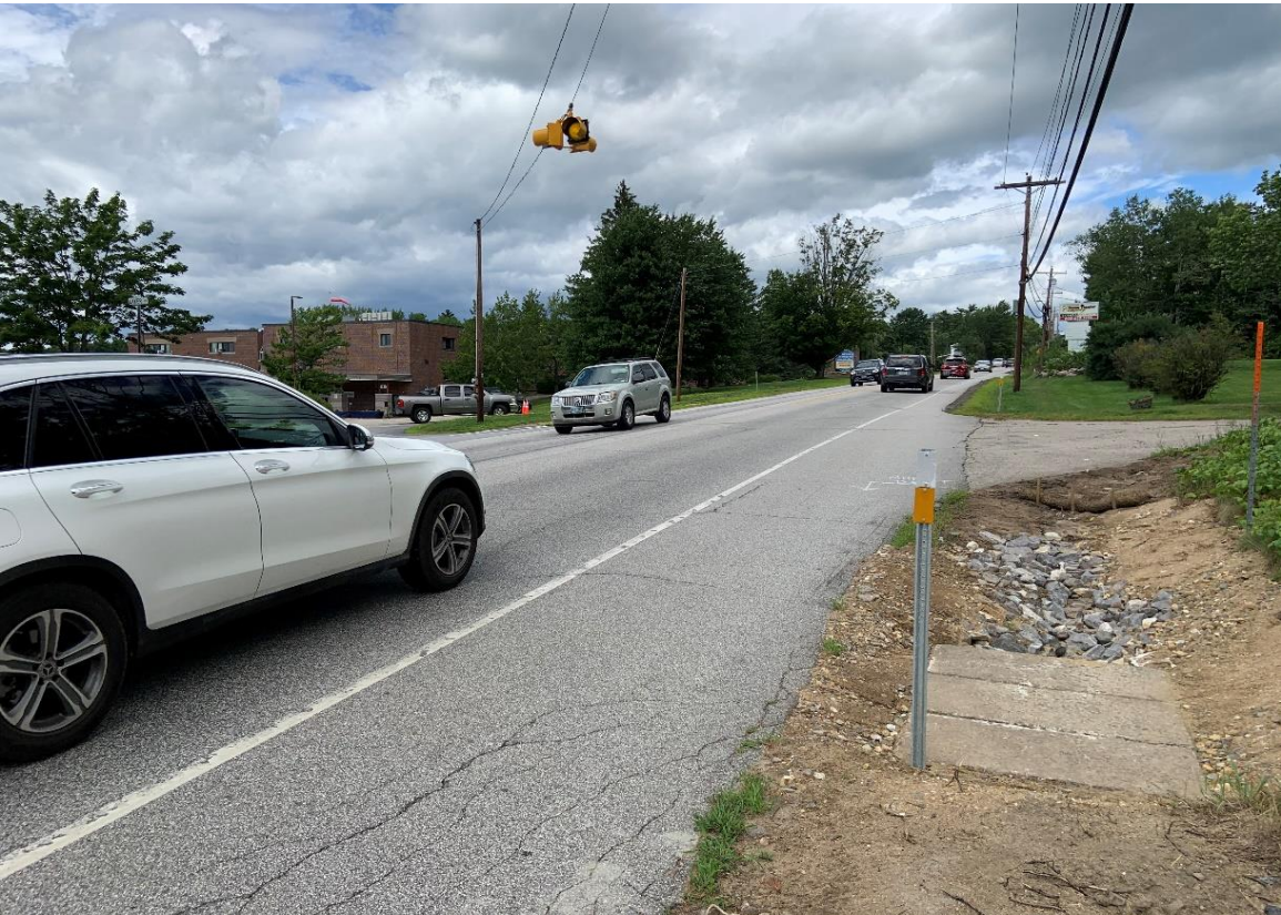
1-B NH Route 25 at Laker Lane (Blinking Signal) facing east
