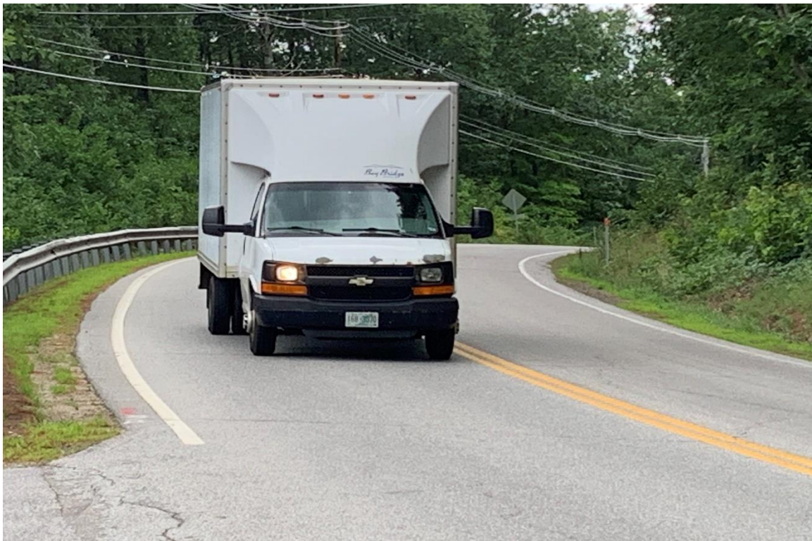
4-B NH Route 25 from patrician Shores intersection. Note poor sight distance facing east. Note sharp horizontal curve.
