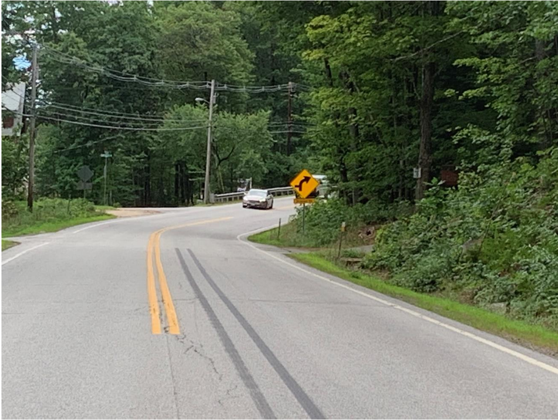
4-A NH Route 25 facing east towards Patrician Shores intersection. Note poor sight distance and inadequate shoulders.
