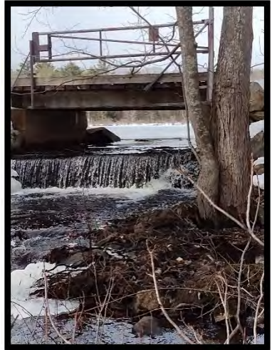
Richardson Pond Dam; Photo Credit: Brian Lenzi
