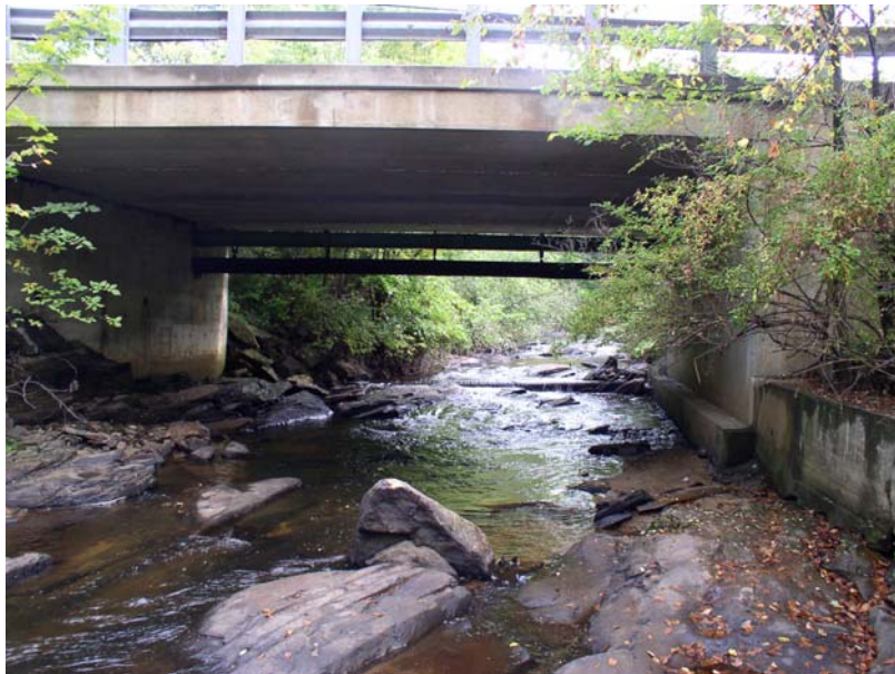
A view of bedrock ledge (and infrastructure) in downtown Belmont.
