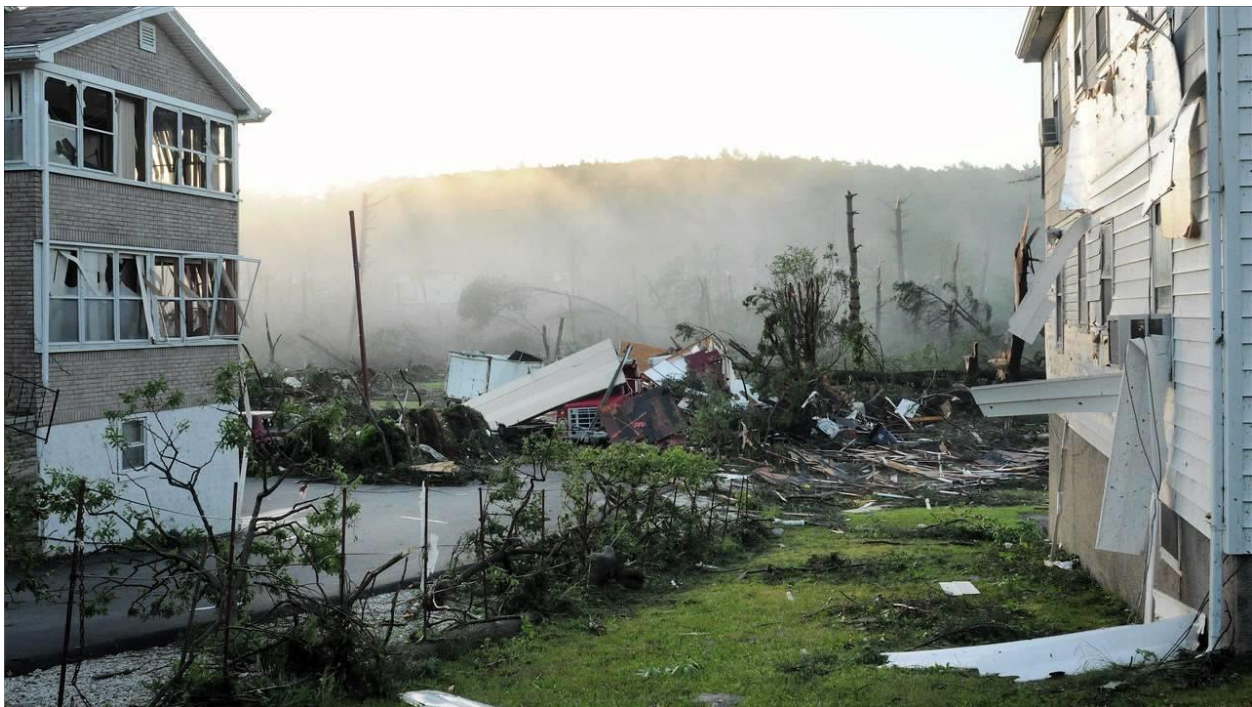
Tornado Damage, Photo courtesy of Fire Chief Normandin
