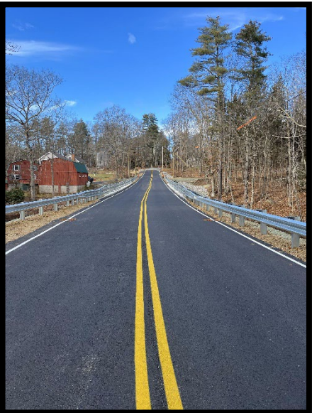
Completed, repaved and striped bridge December, 2023
