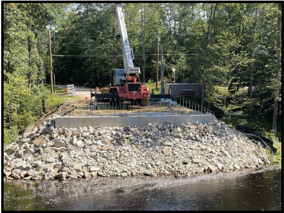
New abutment construction, August 2023
