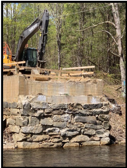
Old abutment during bridge removal
