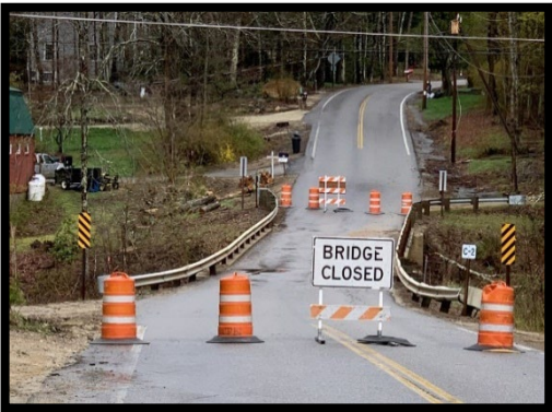
Greenhill Road Bridge, May 2023
