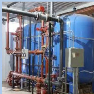
200 gpm Pressure Filter System
