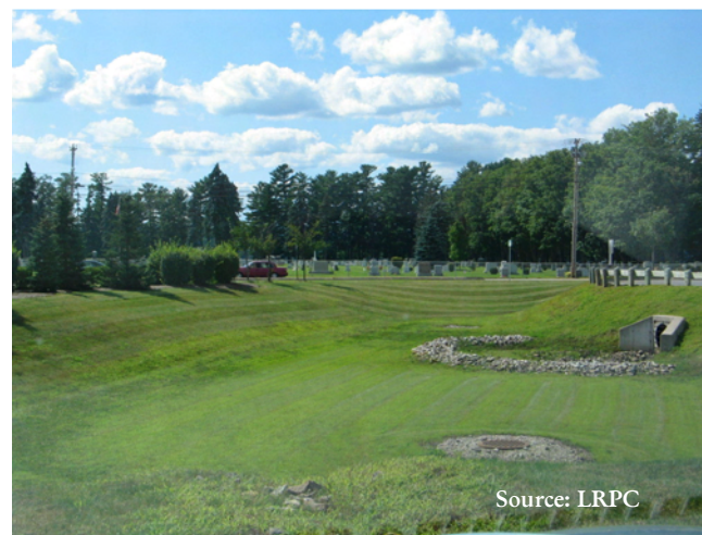
Infiltration basin for large parking area with check dam at inflow
