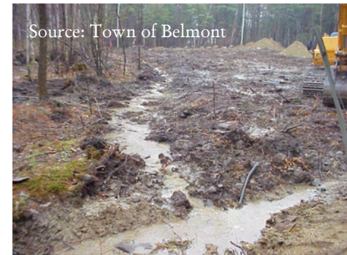
Source: Town of Belmont Construction site with poor/no ESC measures – sites like this can cause many problems off-site as well as on-site.
