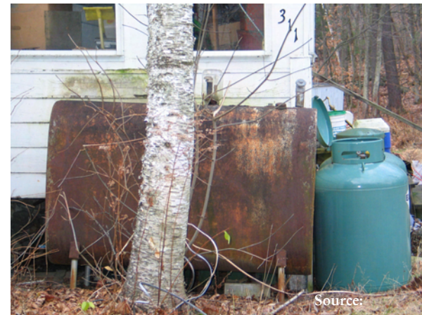
Home heating fuel tanks are unregulated by DES but should be replaced when they become rusty and corroded like the one shown in this picture
