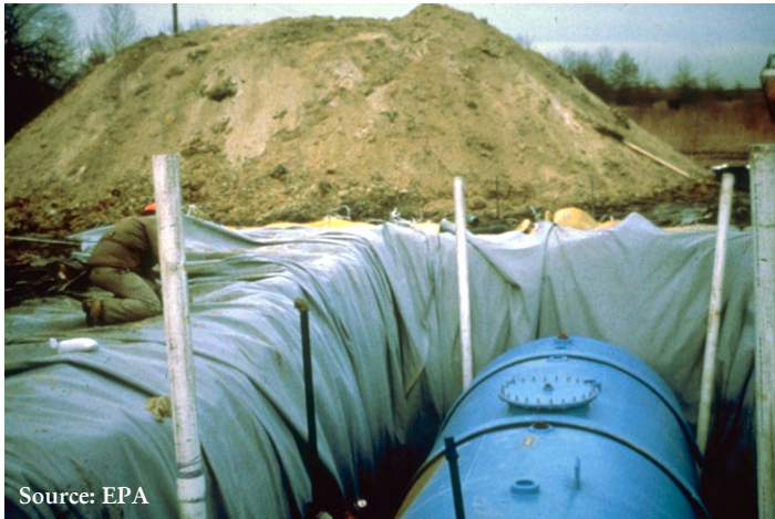
Underground storage tank in lined excavation
