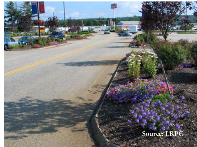
Retrofits to these parking lot islands can create successful bioretention areas
