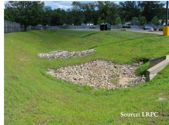
Vegetated swale and check dam used as pretreatment for the infiltration trench
