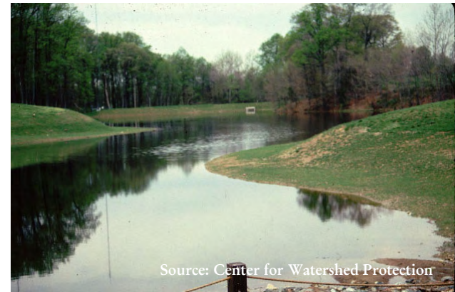
Source: Center for Watershed Protection The shape of this pond is aesthetically pleasing and enhances pollutant removal
