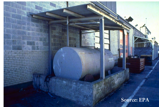
Aboveground storage tank for heating fuel
