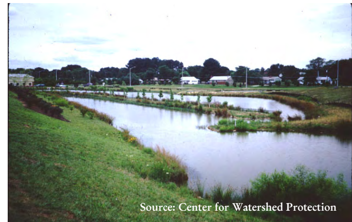
This multiple cell wet pond provides additional treatment pathways while being aesthetically pleasing
