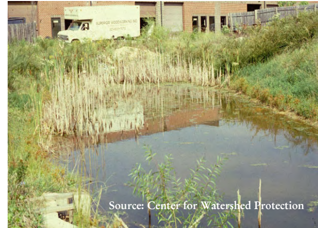
Source: Center for Watershed Protection Infiltration basin clogged due to sediments
