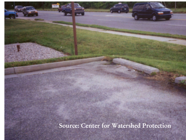
Source: Center for Watershed Protection Infiltration trench next to parking lot with vegetated swale as pretreatment
