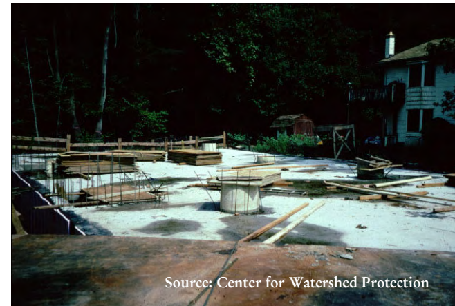
Underground sand filter during construction
