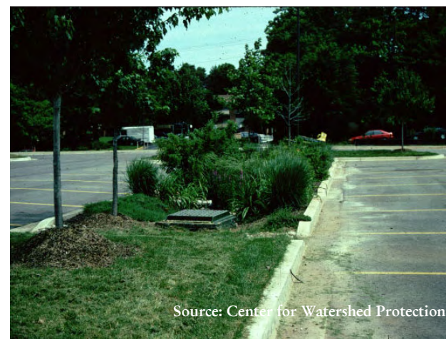
Curb cuts allow runoff to flow from the parking lot into the bioretention area
