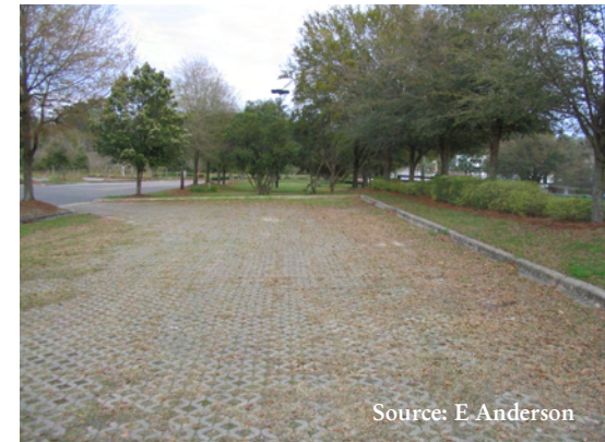
Permeable pavers for overflow parking
