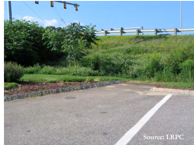
This curb cut directs runoff to a bioretention area
