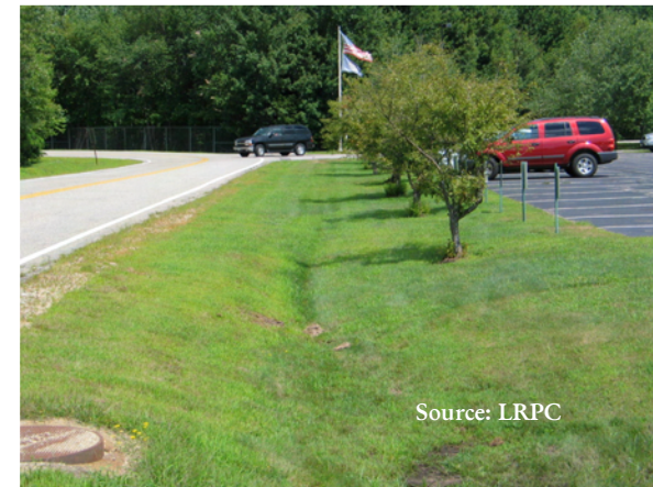
Grass swale used for a road and parking lot
