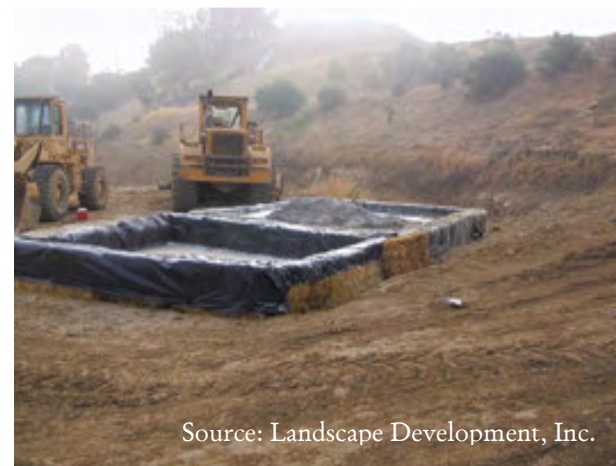
Concrete wash-out station
