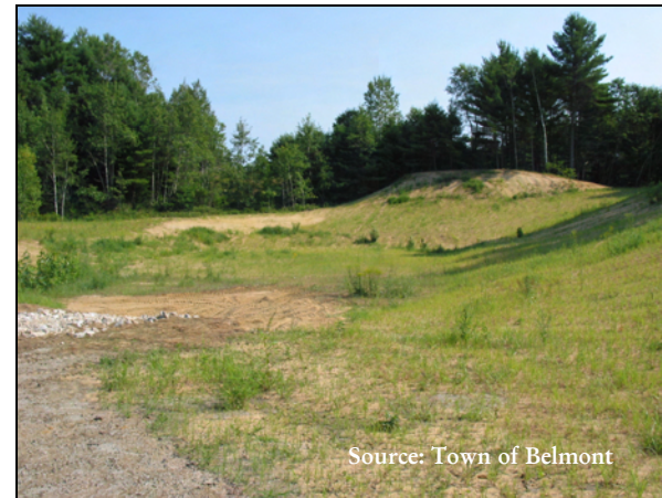
Reclaimed excavation site after seeded with native grasses – no topsoil was used here
