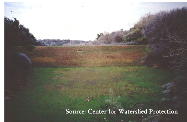
Source: Center for Watershed Protection Dry ED pond for large runoff capacity - lack of woody vegetation on embankments protects structural stability
