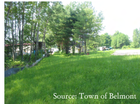
Same parking lot site after seed is established – note silt fence still up to minimize sediment runoff until complete
