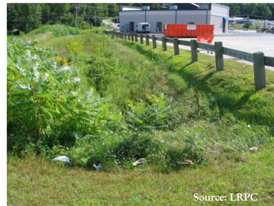
Wet swale adjacent to a commercial parking lot
