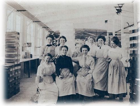
From 1921-1955, the Mill operated as the Belmont Hosiery Company.
