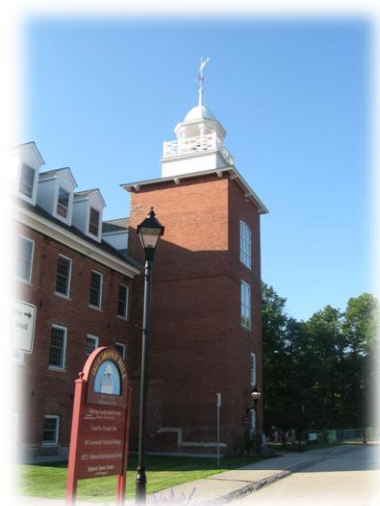
Twenty years after the fire, and 14 years after saving the main building, the Belmont Mill continues to serve the community. Exterior lighting was upgraded to energy efficient LED in 2011 through a federal grant.
