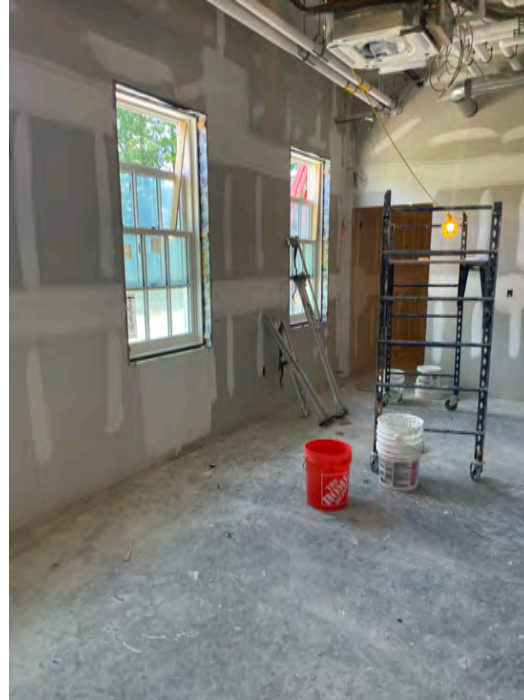
Framing and Drywall for on the Interior of Town Office Building
