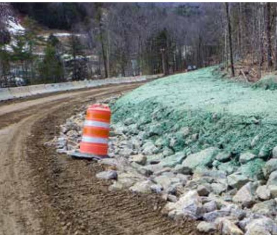
Construction began in December 2017 and will be complete in July 2020. To date the relocation of Houghton Ledge Road is substantially complete with the retaining wall removed and a majority of the steep slope stabilization complete. Drainage replacement and full roadway reconstruction for the 2.1 mile segment will continue through 2018.
