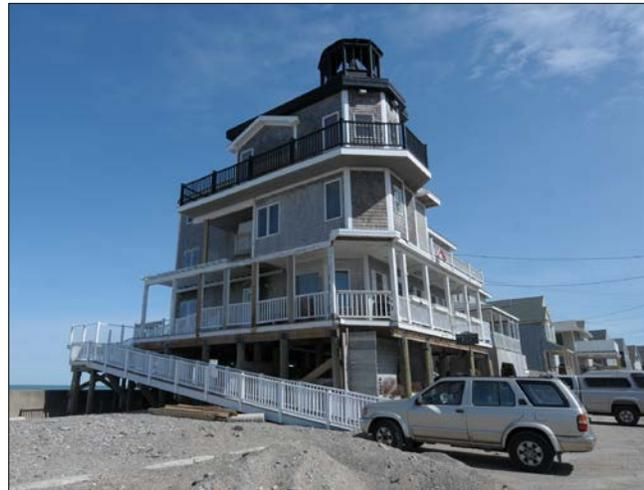
The Ocean Side Inn in Scituate, MA was elevated in 2010 to protect against significant damages. FEMA Photo
