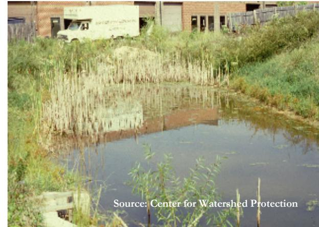
**Infiltration basin clogged due to sediments**
