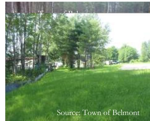
Same parking lot site after seed establishment – note silt fence still in place to minimize sediment runoff until complete
