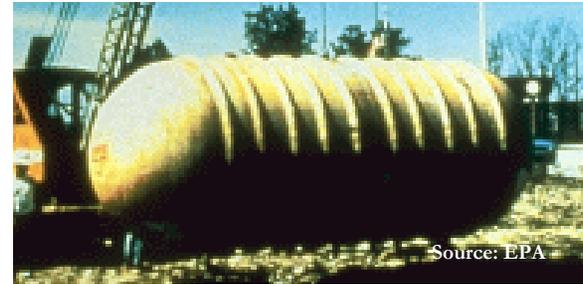
UST – Fiberglass Reinforced Plastic Tank
