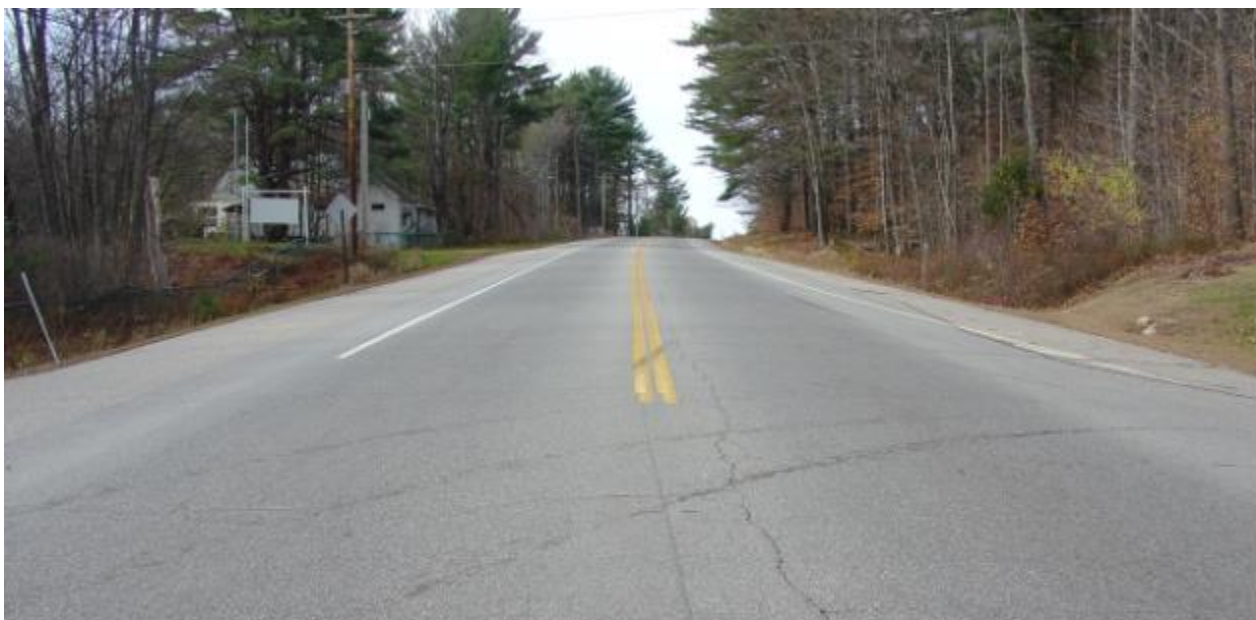
Existing conditions looking west on NH Route 104 from the centerline between Meredith Woods RV Park and Clearwater Campgrounds
