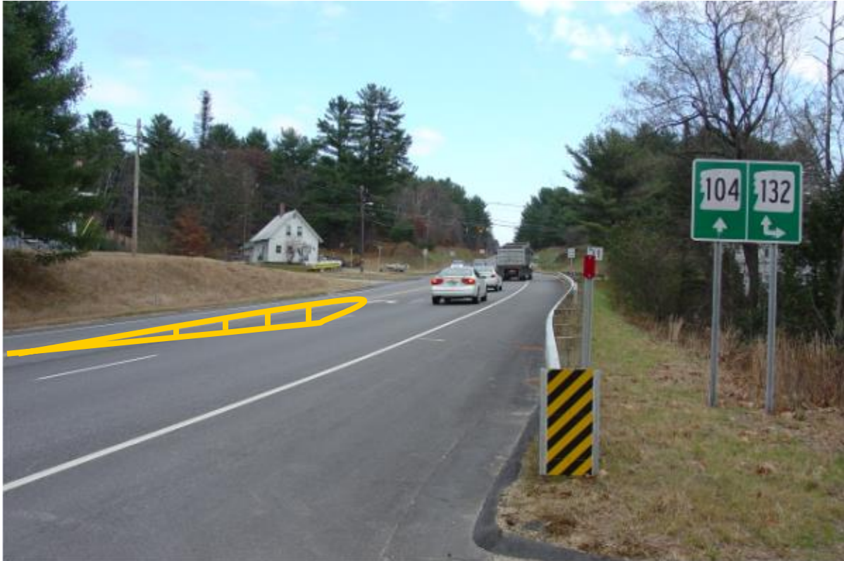
NH Route 104 at Main Street and Firehouse Lane – Potential Striping Improvement Concept
