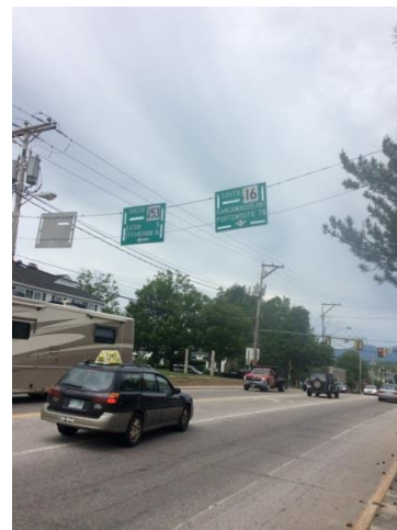
Figure 10: NH16 / NH113 headed west towards NH 153
