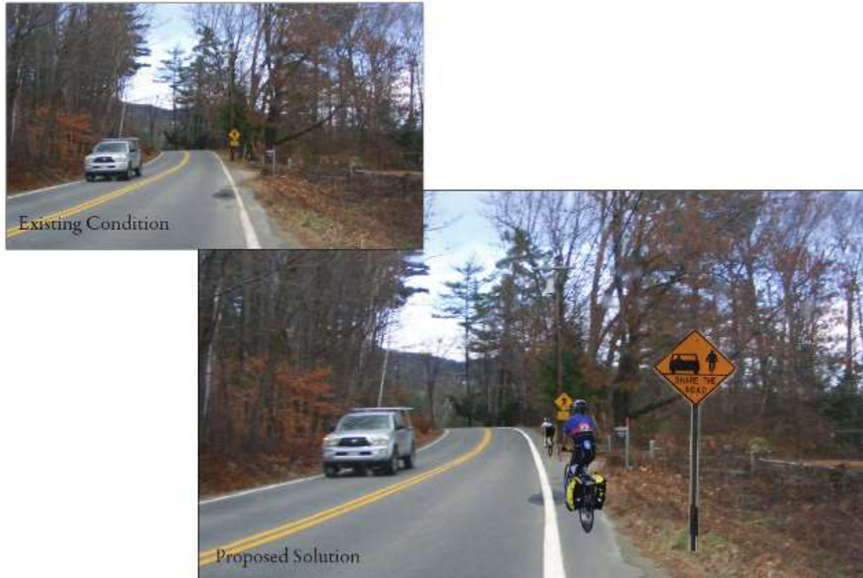
Figure 10: Conceptual rendering of a lane width modification along NH Route 113 in Holderness. Existing 11½ - 12 foot lane is shown above. Proposed solution with 10½ - 11 foot lane using existing pavement is shown below, with added Share the Road signage. 8
