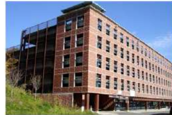
Brattleboro's new transportation center helps connect a small town with the surrounding region. (US EPA)
