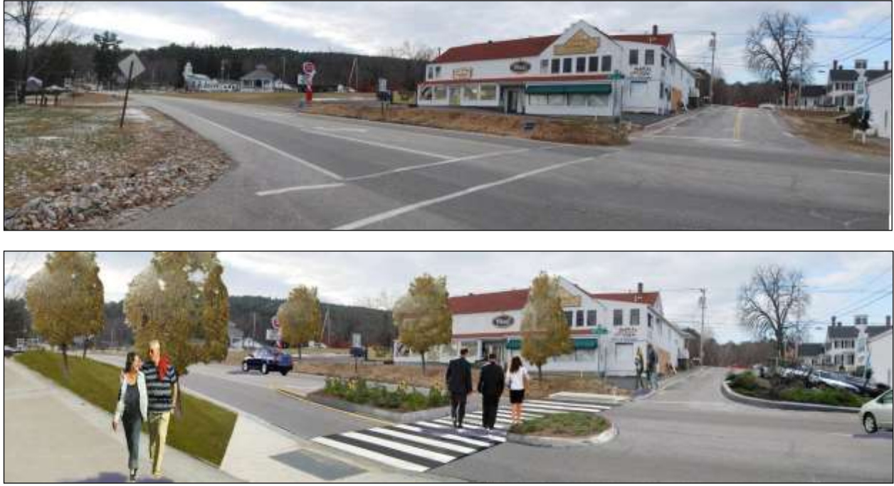
Figure 11: NH Route 25/Lake Street Intersection (Looking West) – Current (top) and Proposed Improvements (bottom) 9
