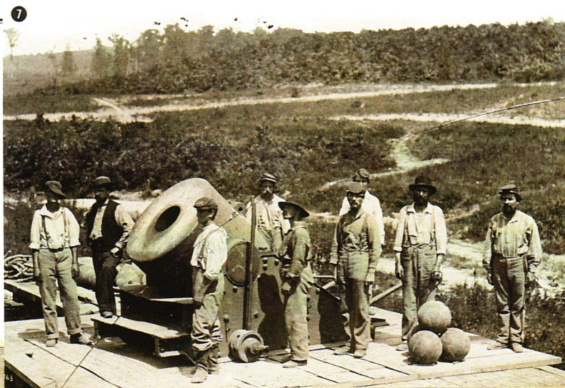
7 SERVING THE DICTATOR Federal gunners attend a monstrous mortar called the Dictator, used during the siege of Petersburg. Transported along the tracks of the City Point Railroad and a military railway nearby, the 12-inch mortar could hurl a 200-pound shell more than two miles.
