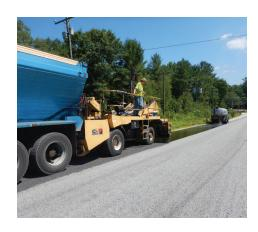
provide increased durability and are typically applied to roads with traffic volumes up to 2,500 AADT.
