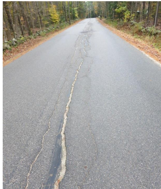
An example of Longitudinal Cracking
