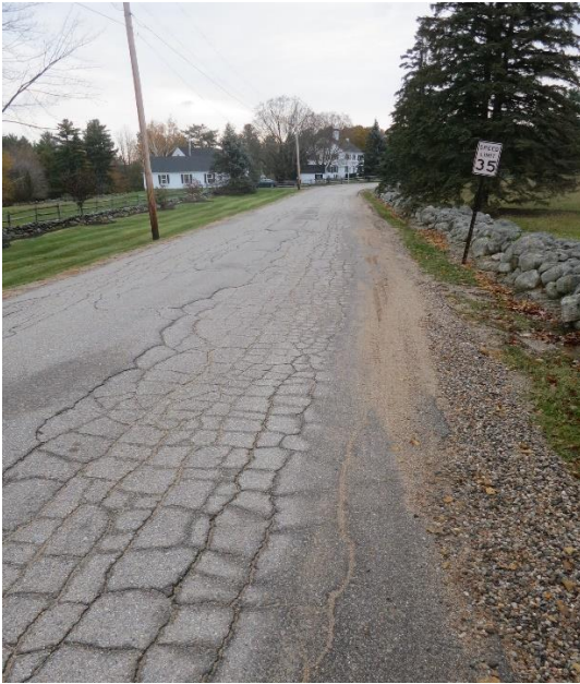
An example of Alligator Cracking
