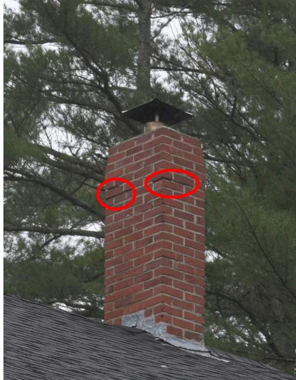
Figure 60: Mortar loss at east chimney
