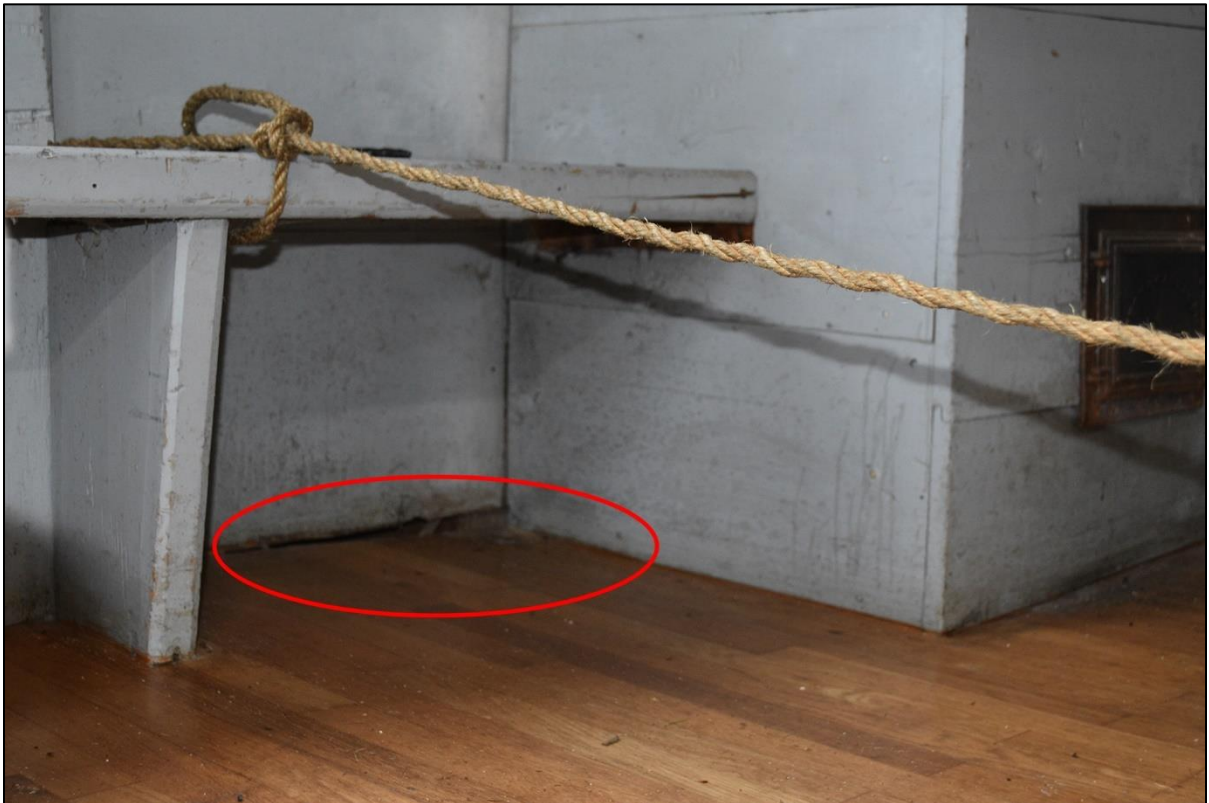
Figure 63: Gap between floor and wainscot where chimney has pulled down adjacent floor as it has settled
