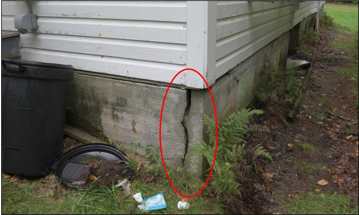
Figure 64: Crack at northeast corner of 1934 privy addition
