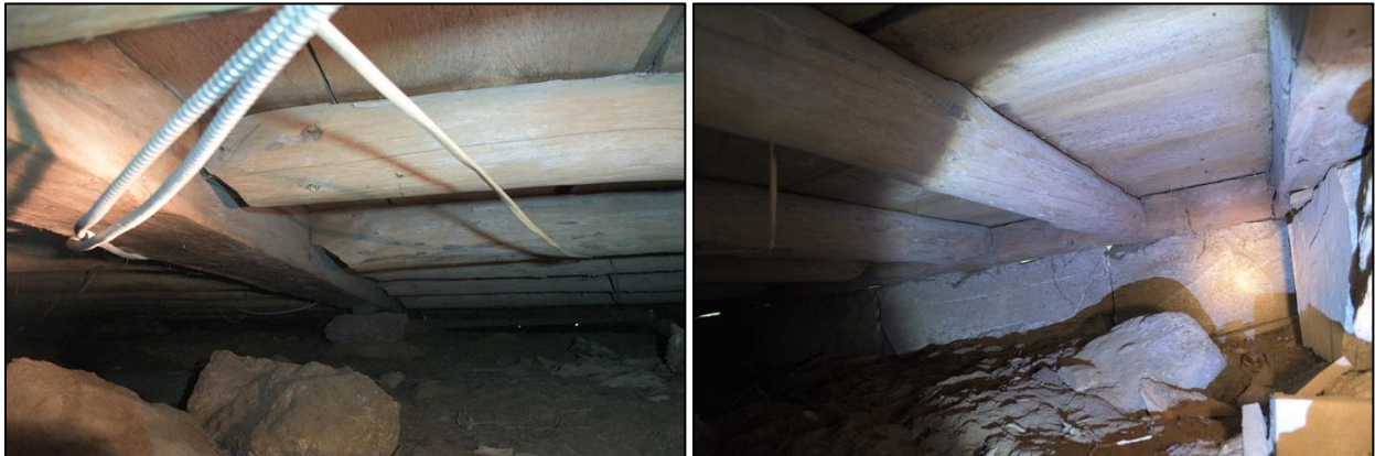
Figures 28 & 29: Views in crawlspace beneath main block. Left: facing slightly east of south, toward Town House door with heavy cellar girt at left and half-round floor joists. Right: facing west, toward corner of building showing exterior wall.
