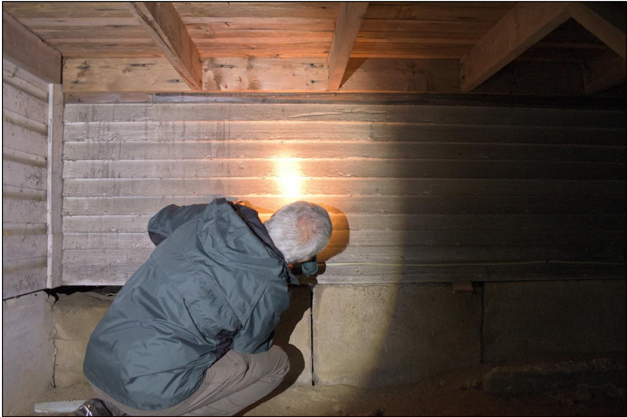
Figure 27: Area beneath stage with 1934 privy addition at left (note novelty siding) and original 1798 clapboards at original north exterior wall of main block.
