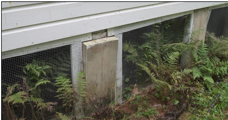
Figure 65: Slipped concrete pier beneath kitchen/stage addition
