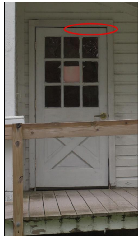
Figure 59: ADA entrance at east elevation, showing gap at top of door
