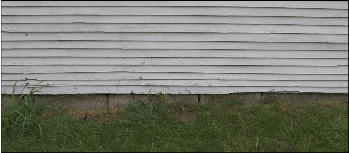
Figure 58: Detail of west elevation, showing grass against the foundation and walls of the Town House
