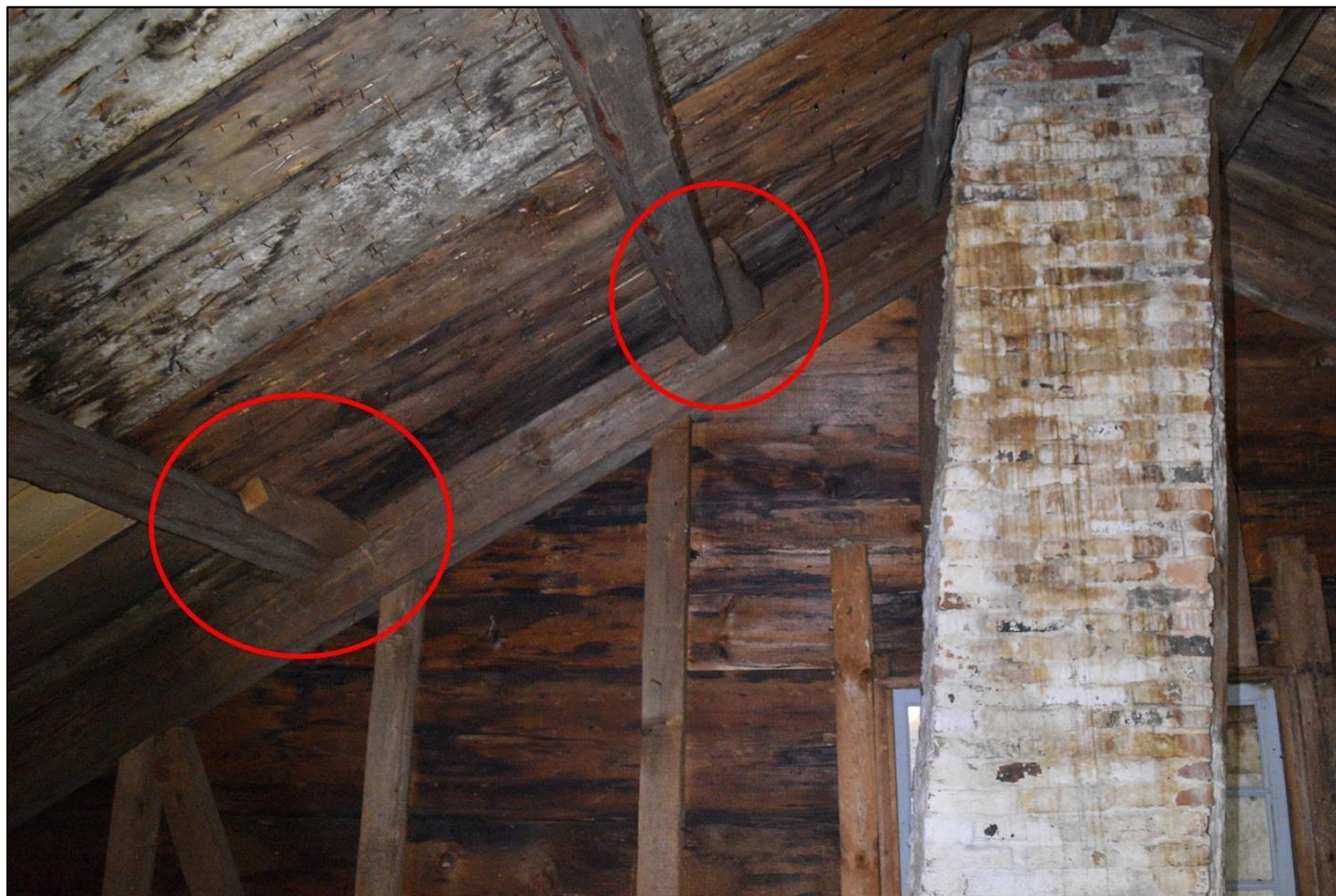
Figure 51: Blocking at west gable end added in the 1870s to extend the eaves as part of the building renovation
