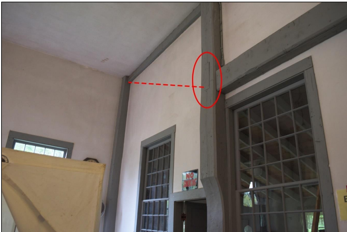
Figure 35: Infilled mortise that once held up the front of the gallery seating and approximate angle of gallery floor (northwest corner of hall)
