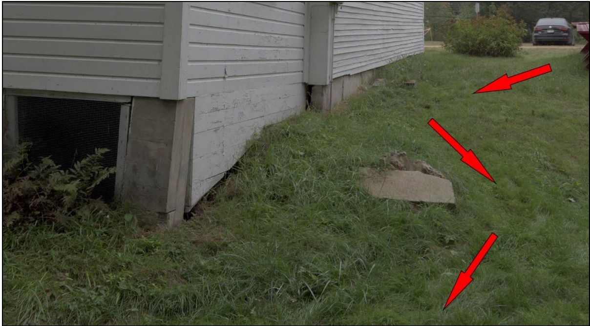
Figure 54: Slope at west side of Town House (from north). The arrows indicate the flow of surface run-off
