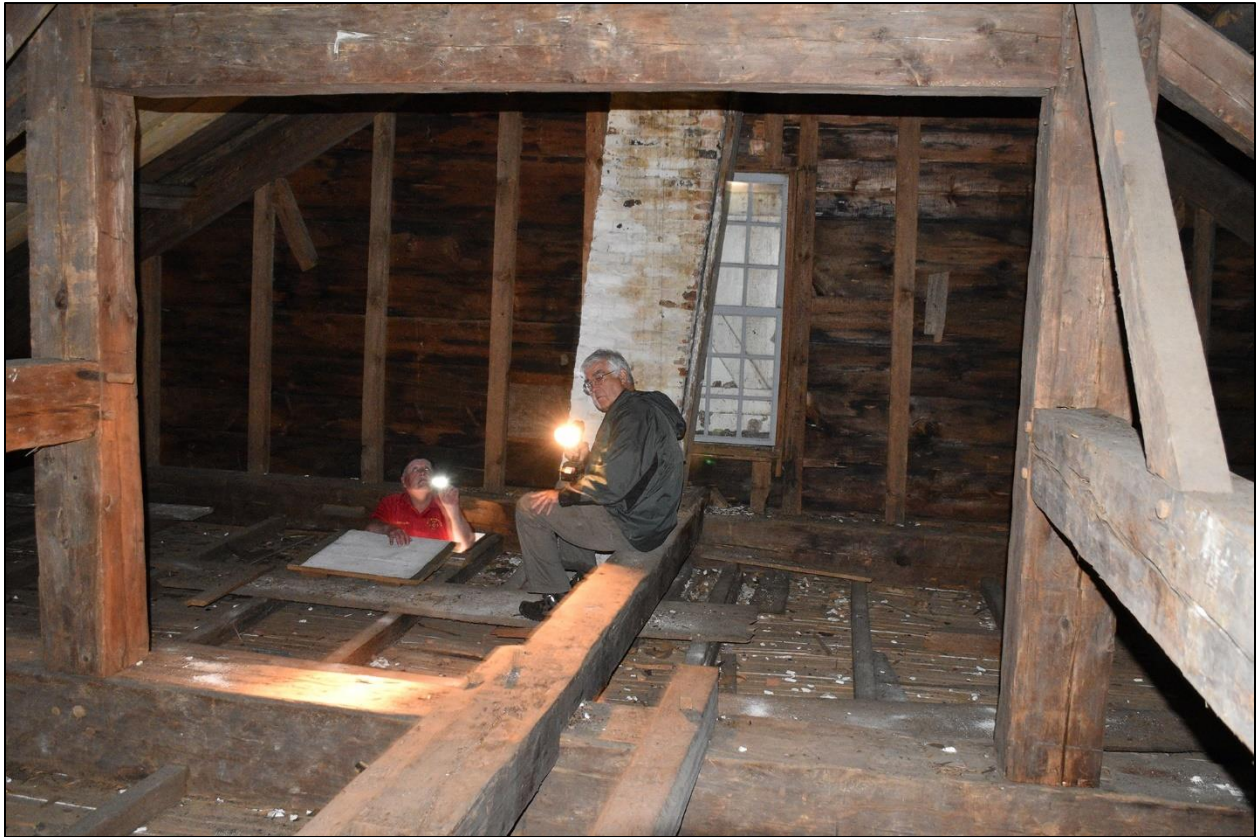
Figure 52: West gable end of New Hampton Town House (note that the chimney was constructed on an angle)
