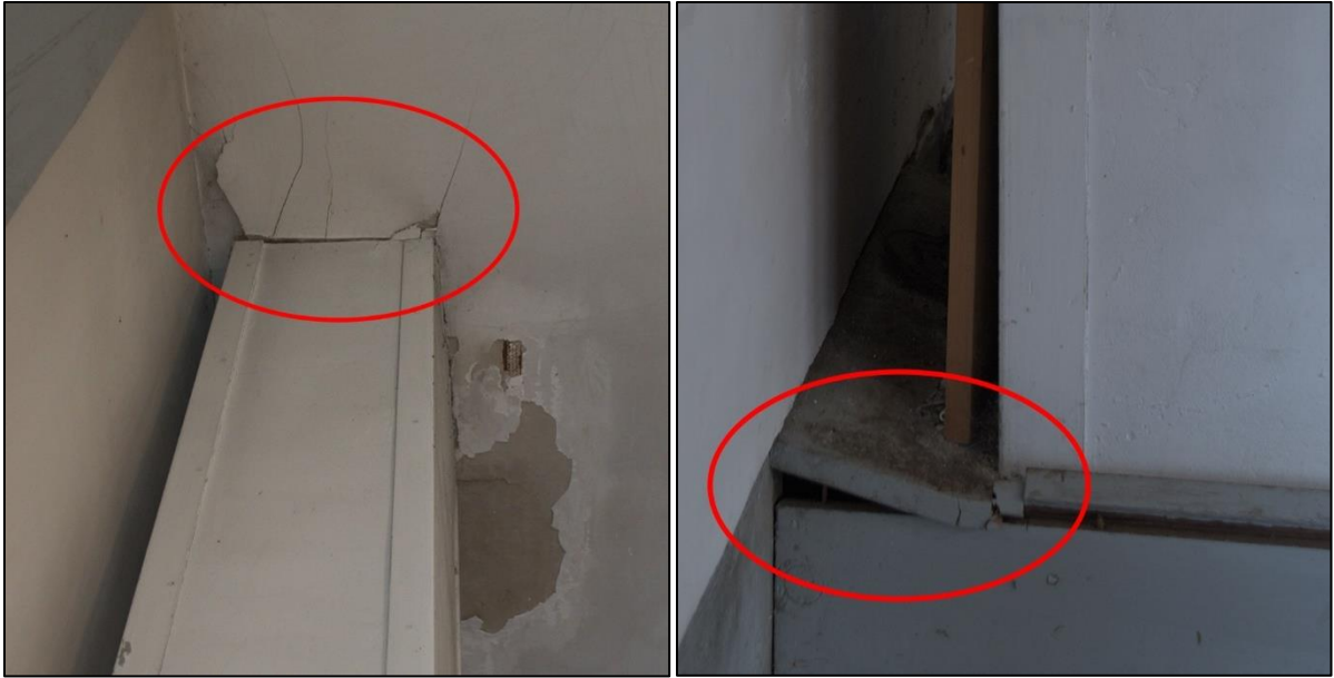
Figures 61 & 62: Damage to ceiling adjacent to top of west ceiling caused by settling of the chimney stack (left); and at intersection with wainscot (right)
