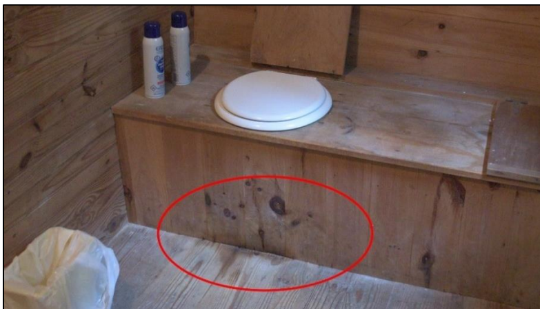
Figure 68: Staining of porous wooden surface in privy
