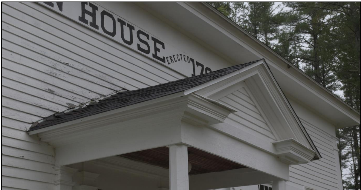
Figure 57: Detail of south elevation, showing paint loss over entrance portico
