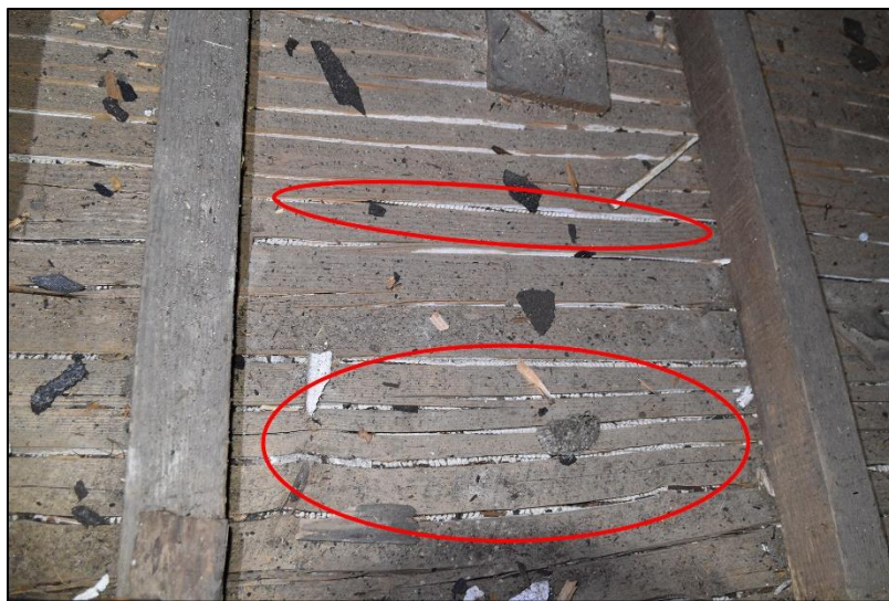
Figure 50: 20 th century metal lath (circled) between original 1798 split-board lath
