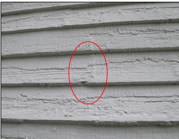
Figure 20: Skived and lapped original clapboards
