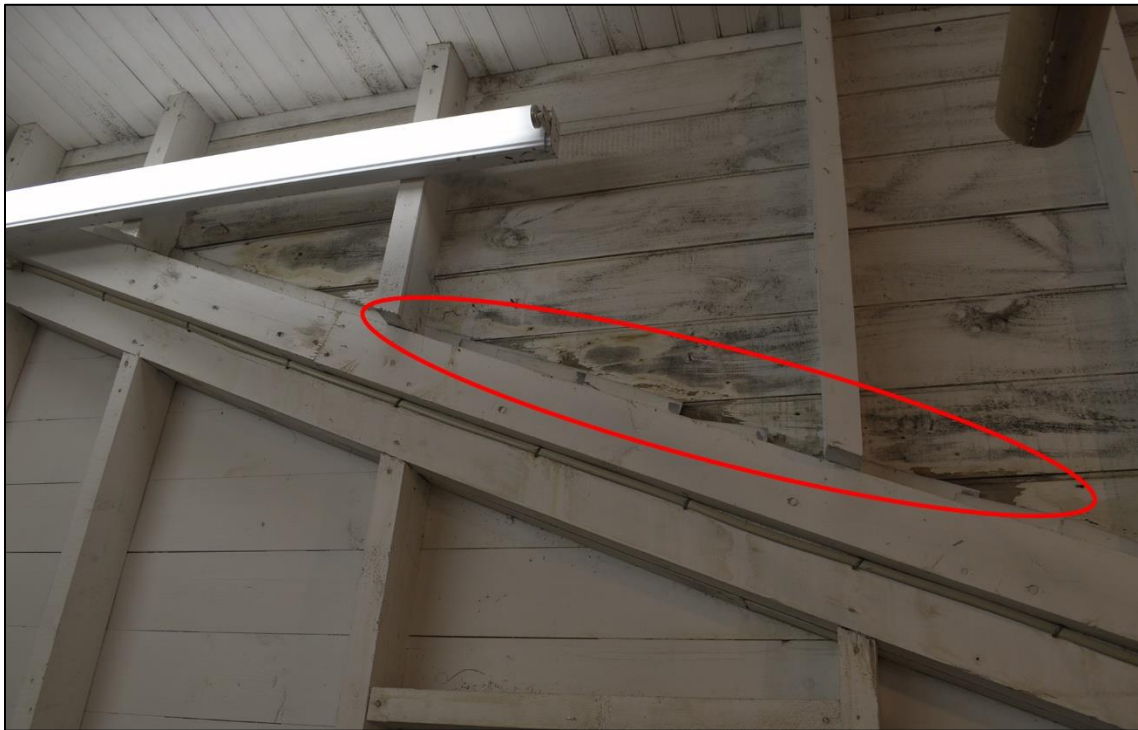
Figure 70: Signs of rot and mildew/water-staining on west stage side-wall at intersection with kitchen roof
