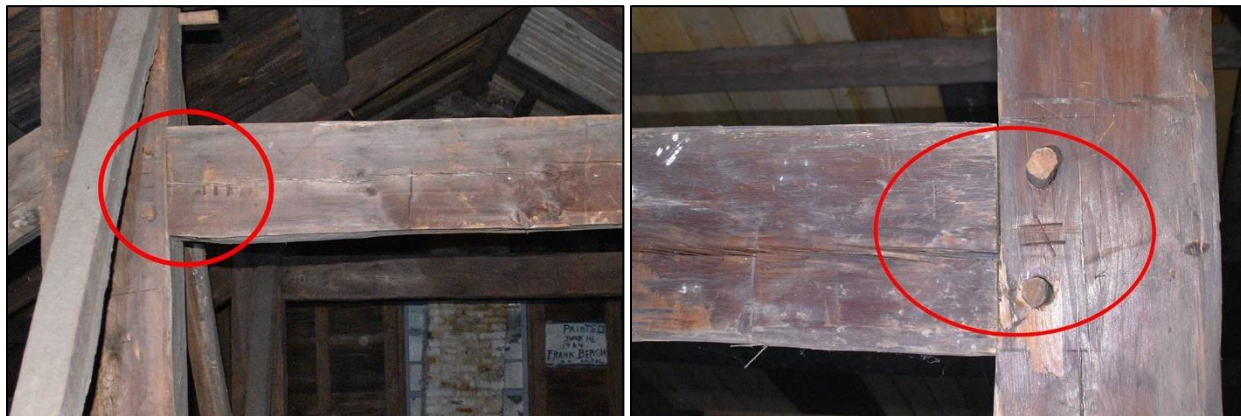
Figures 48 & 49: Samuel Kelly, Jr.'s "marriage marks" are clearly visible at the attic frame
