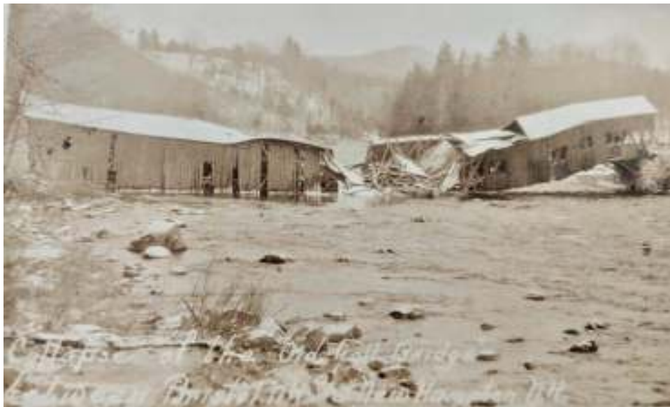
Collapse of a Toll Bridge (built after Capt. Smith's)
