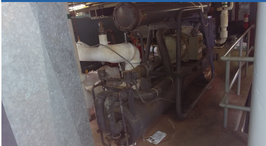
Failing chiller unit dating back to 1961 - beyond repair.
