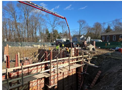
Photos of some of the work completed for the new Library project at 1 School St. The first photo shows wall panel construction, and the second shows concrete poured into the wall foundation forms.
