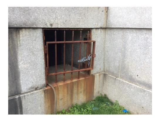
The metal grate underneath the front staircase has rusted to the point of warping the metal. It can no longer close. A chain holds the grate in place, but this clearly needs to be replaced. The rusted metal has also discolored the stone underneath where the grate sits.
