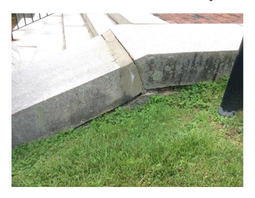
Under the front stairs, wear on the stone that connects to the ground is evident. The stairs are secure for use, but weather has caused the stonework to erode over time. This needs attention.
