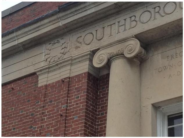
Weather has caused the "S" and "O" on the front stone work of the library's sign to erode over time. There is also assorted discoloration and "white lines" that appear through the stone.
